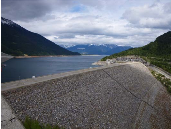
Mica Generating Station
