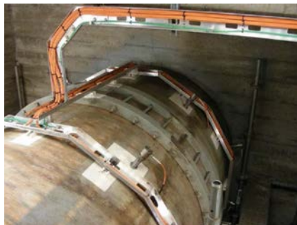
Flowmeter Layout PIV4 Cable Tray
