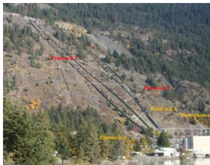
Bridge River 1 - Penstocks
