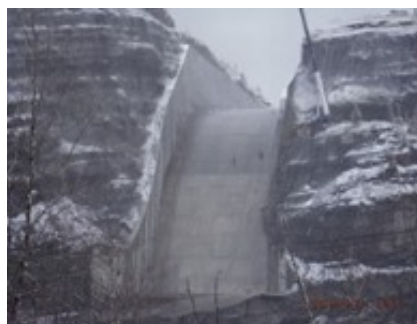
WAC Bennett Dam Spillway Chute – completed, September 2016
