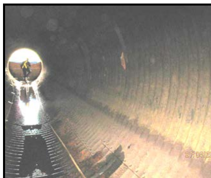
Wahleach – tailrace tunnel, steel section
