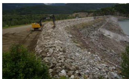
Restoration of the upstream rip rap
