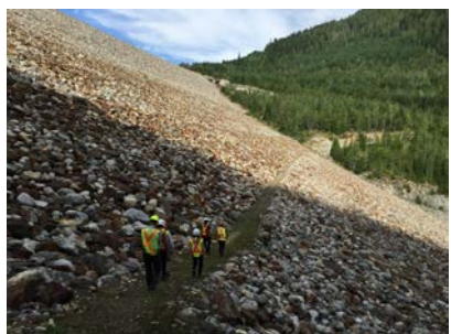
Mica Dam – downstream slope
