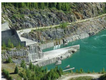
Spillway and Outlet Works Flip Bucket
