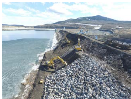
Start of rip rap placement from left side of dam, March 2017
