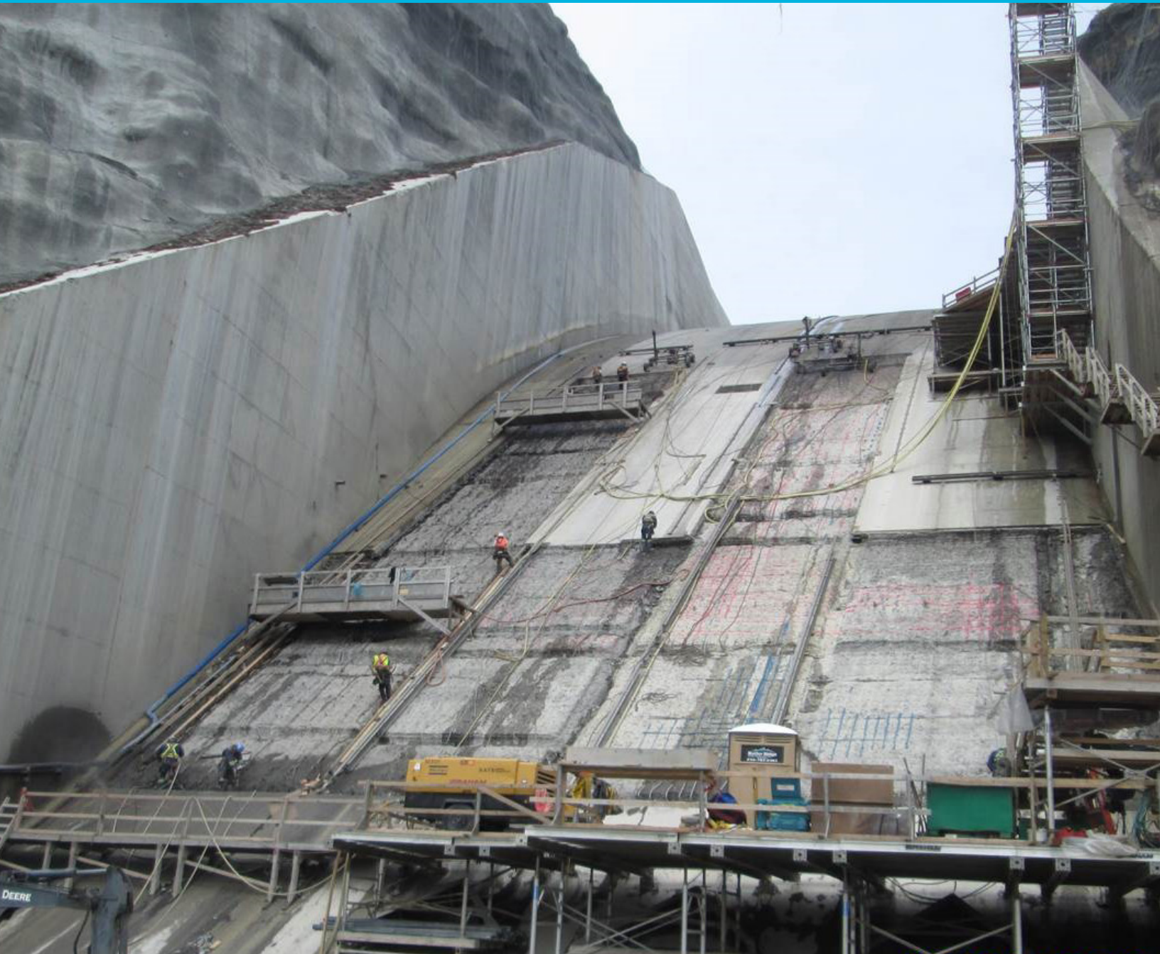
2016 spillway repairs at WAC Bennett Dam
