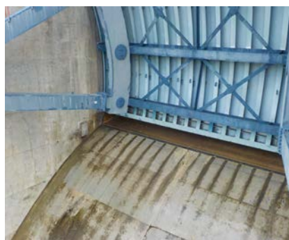
Peace Canyon Spillway Gate
