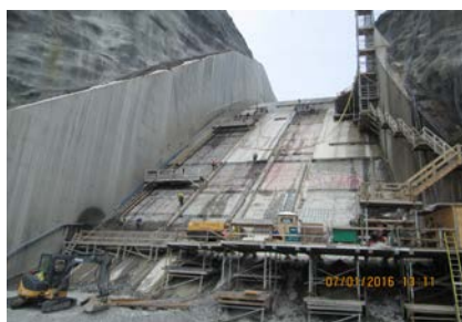
Resurfacing of lower portion of spillway chute, July 2016
