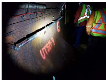
Wahleach, UT-SM9 at the Upper Tunnel lining break.
