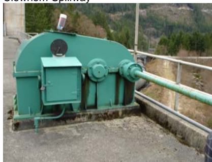
Clowhom Spillway- Equipment
