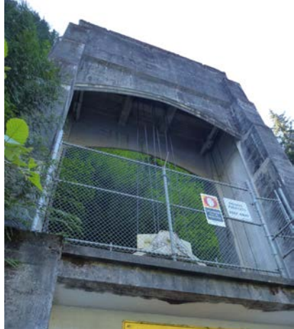
Alouette Headworks Tower
