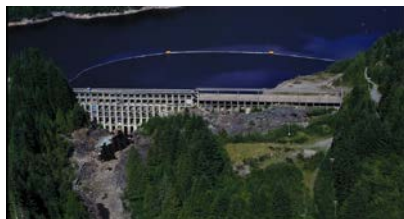
Jordan River Diversion Dam
