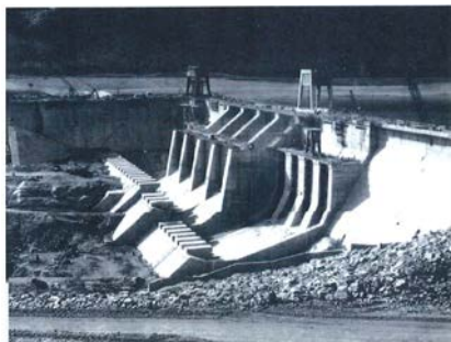
Hugh Keenleyside Low-Level Outlets (right side of photo, taken after construction)
