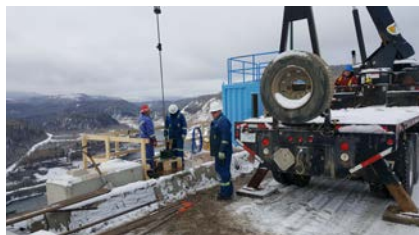
Investigating unplugging techniques for cross-arm device
