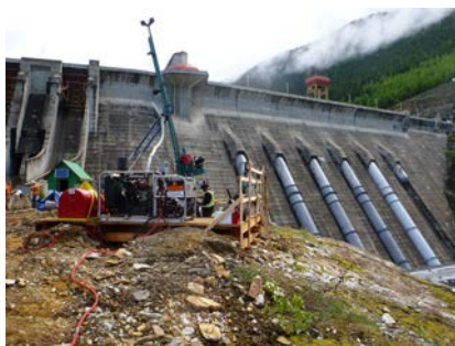
Drilling in the Marble Shear Block
