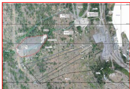
Aerial view of the Bridge powerhouses and penstock slopes
