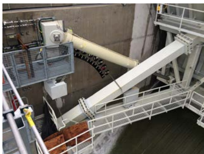
New Spillway Gates
