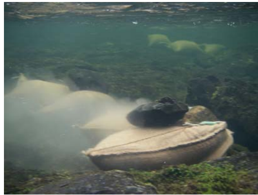
Figures 4a and 4b. Application crew securing pollock filled burlap bags to the bottom of the river using large cobbles.
