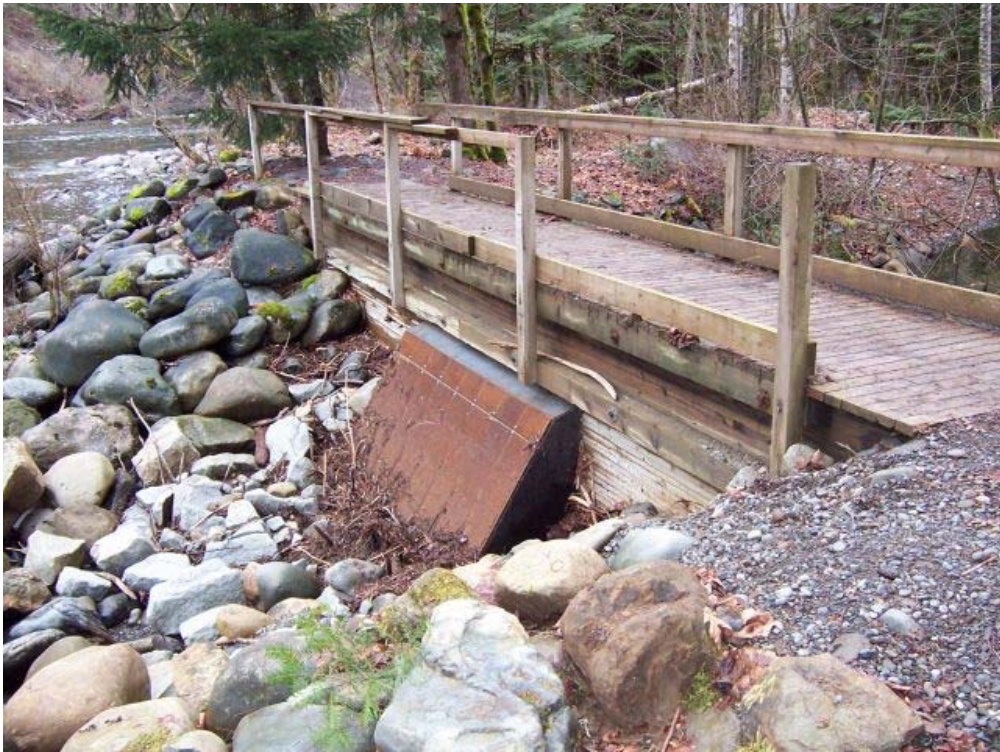
Figure 5. Powerhouse side-channel footbridge with screened bank intake in place.
