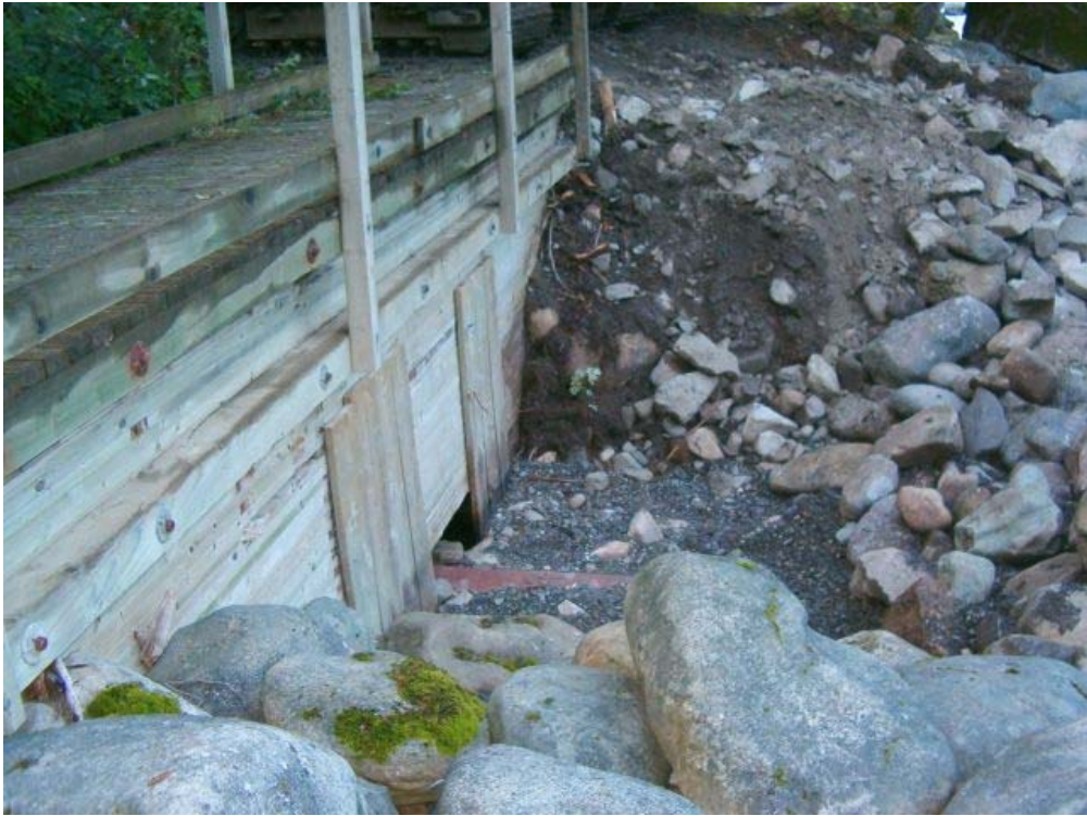
Figure 4. Replacement of inlet channel with pipeline (seen in centre of photo).
