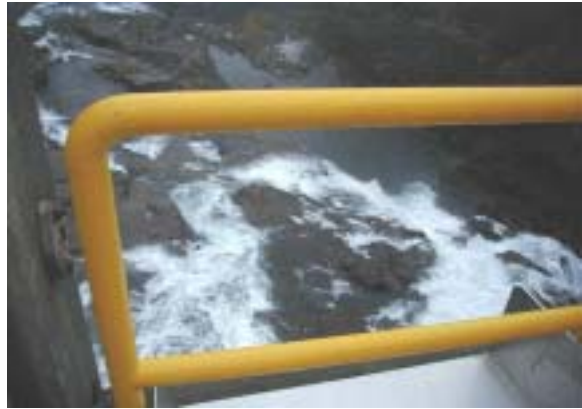
John Hart Dam Spill/distribution Location
