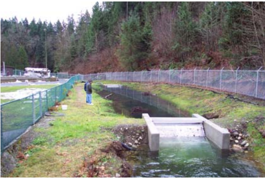
Figure 7 – Jack Creek Rearing Channel at Puntledge Hatchery
