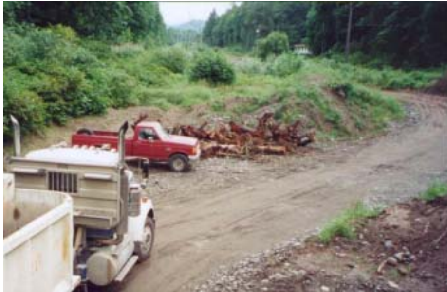
Figure 3. Early in construction just north of the transmission line tower.
