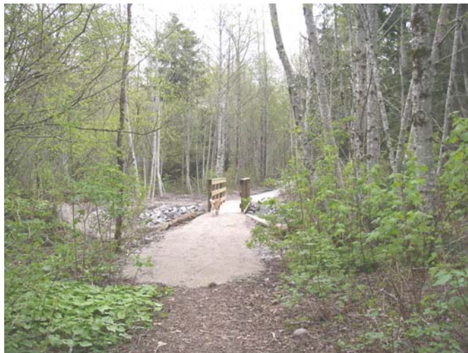
The final bridge installation adjacent to the WestBarr Logsort Road
