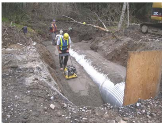
Installing the culvert
