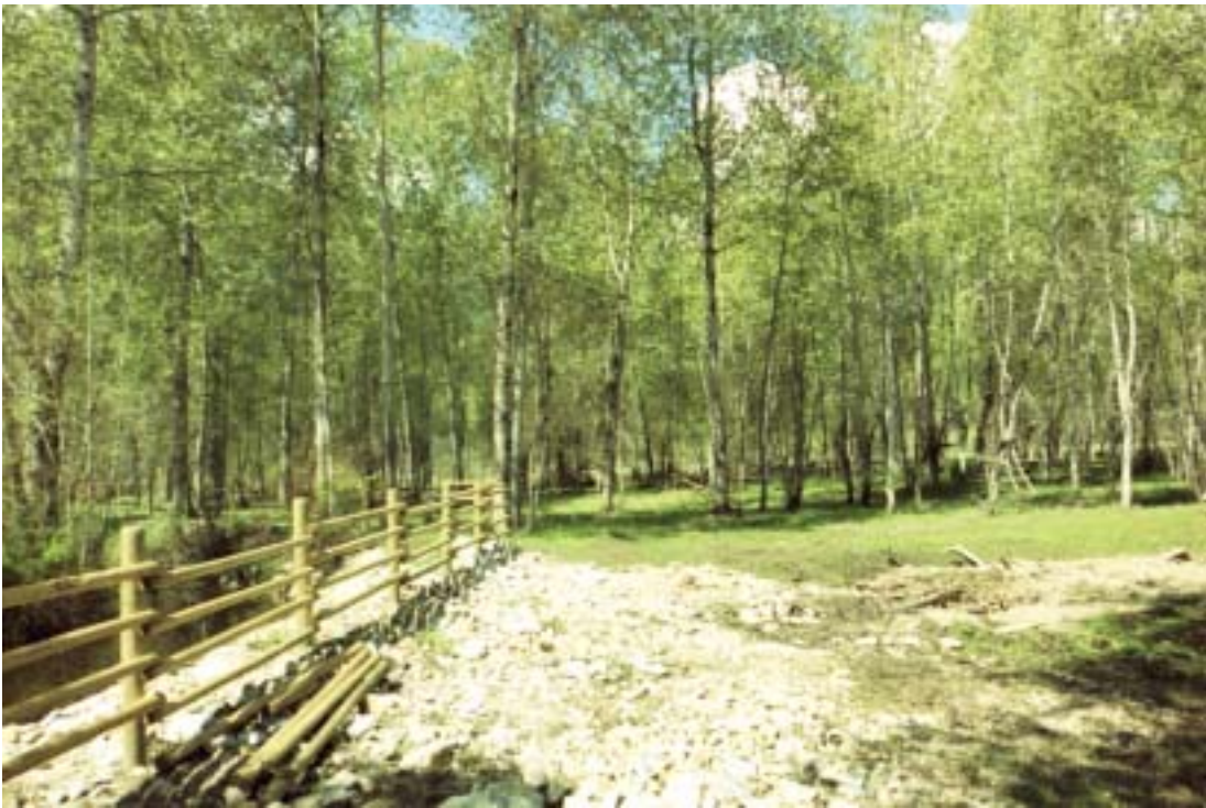
After 29: The bank at the corner is armoured and the scour hole filled.
