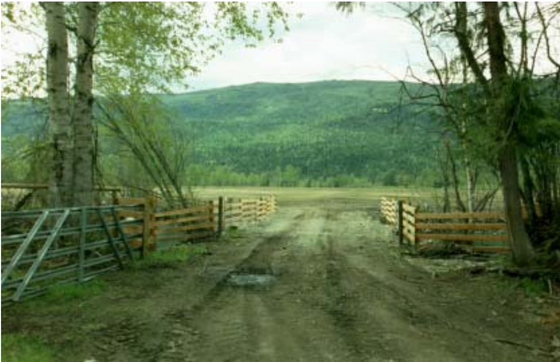
After 10: Two culverts have been placed and the riparian area fenced.
