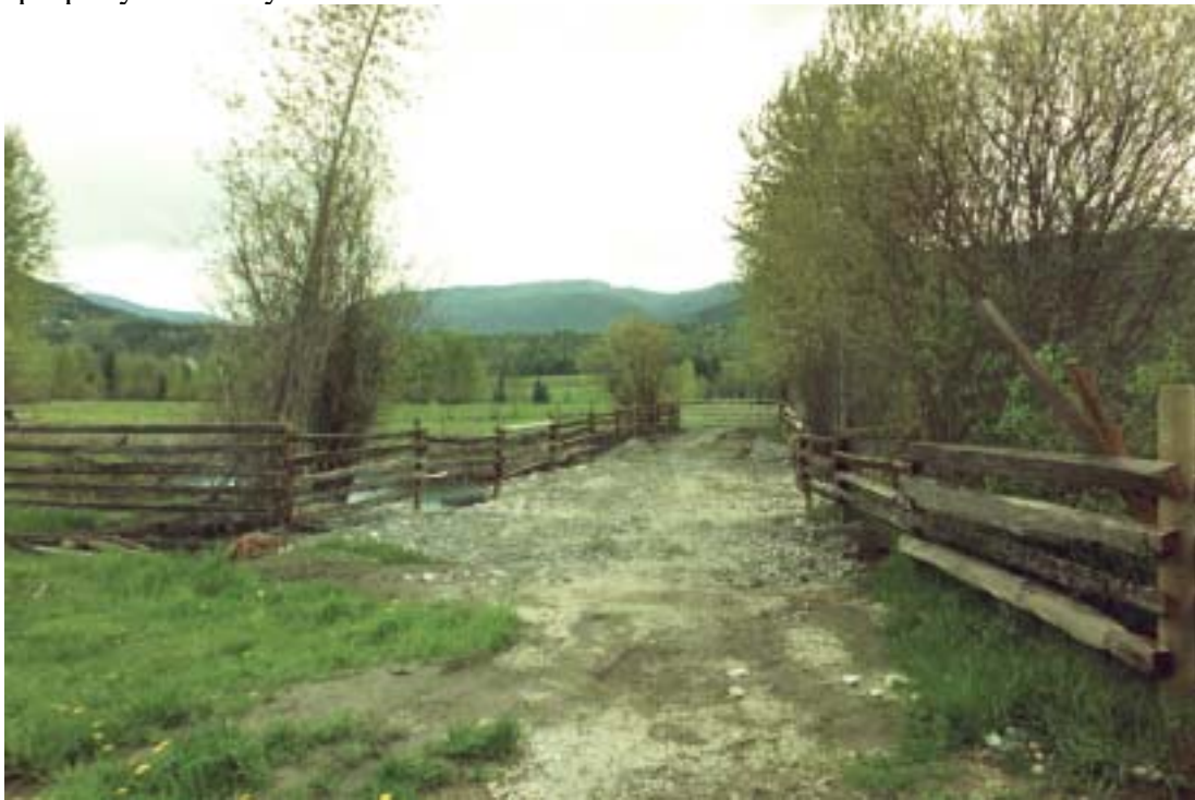
After 15: Culverts have been added and the crossing graveled and fenced.
