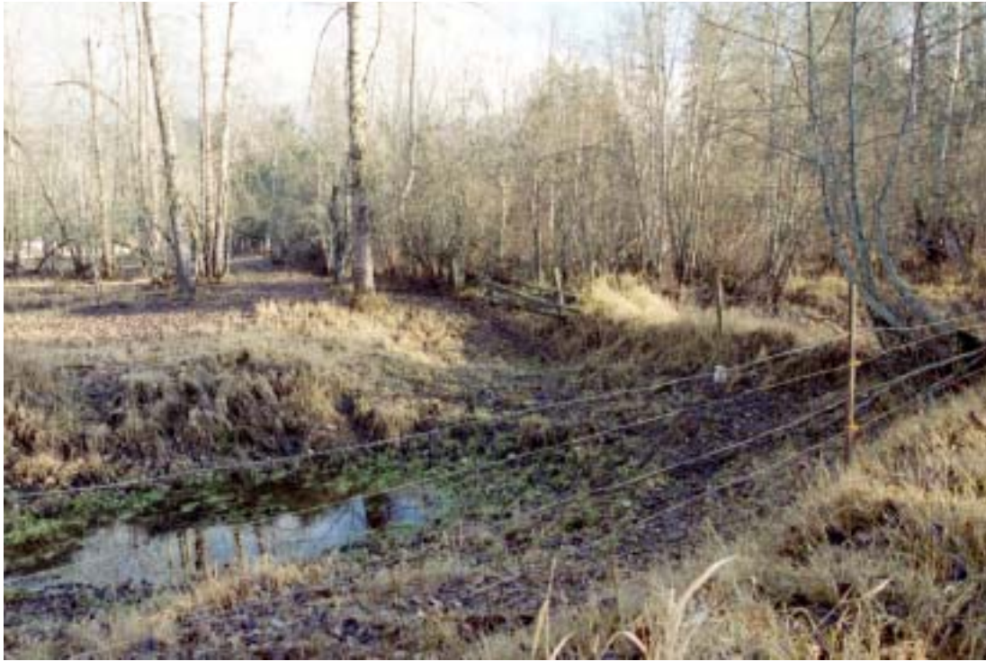
Before 30: A different view of the hole scoured on the backside of the 90 0 corner on the Huwer property.
