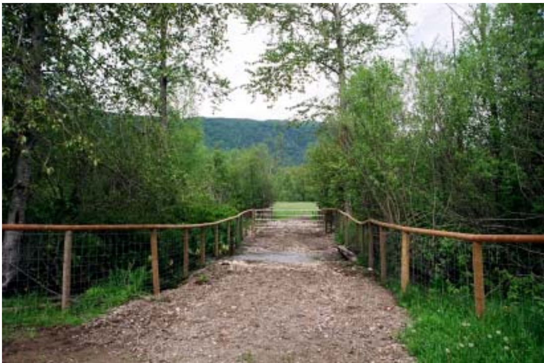
After 9: The access point has been rocked, graveled and fenced.
