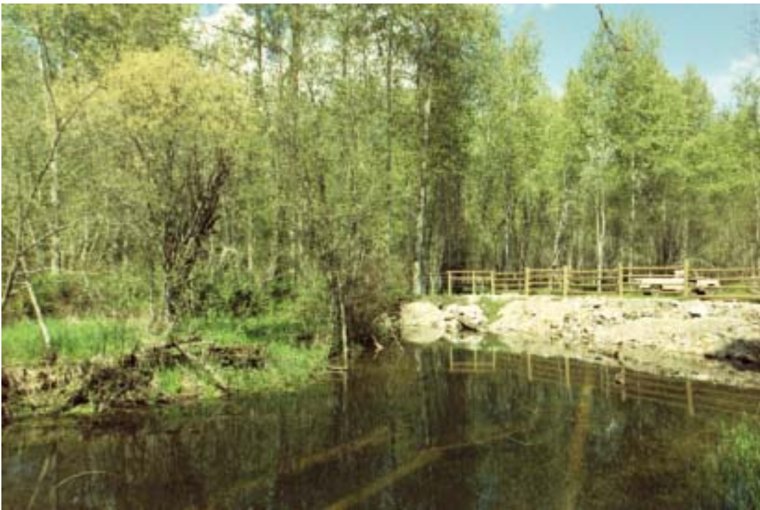
After 28: The corner was rounded and armoured to prevent erosion.
