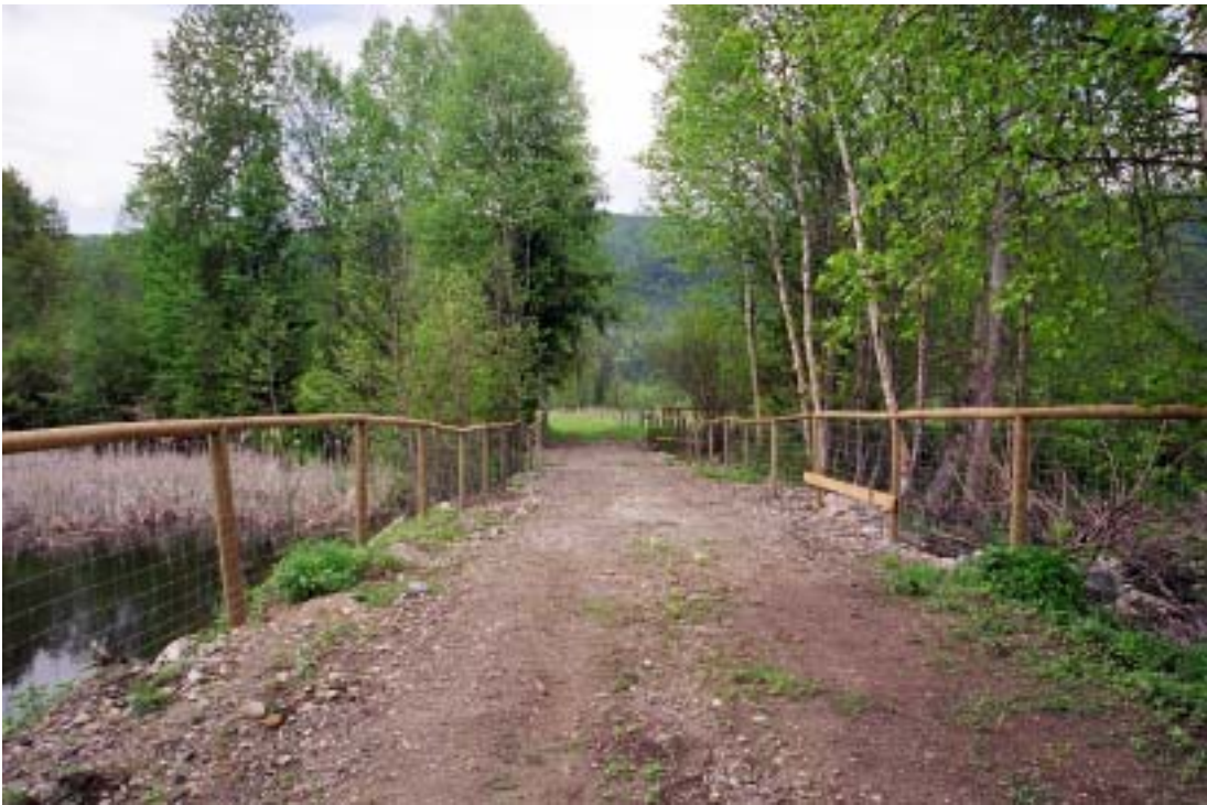
After 7: The same view as above with the bridge replaced by a culvert.
