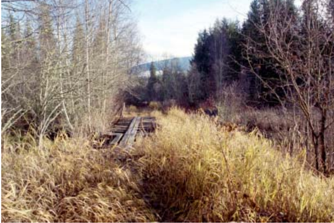
Before 8: Looking eastward across the old bridge.
