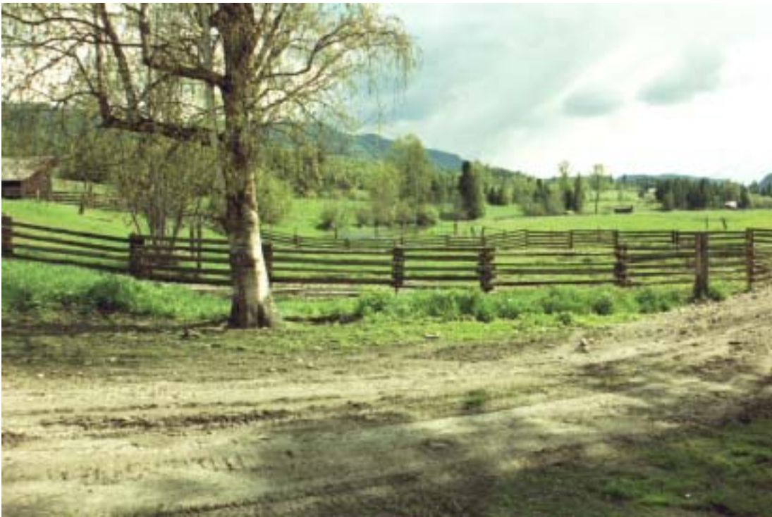
After 18: The road has been upgraded and the fence rebuilt to keep cattle from entering the water and trampling the stream banks.
