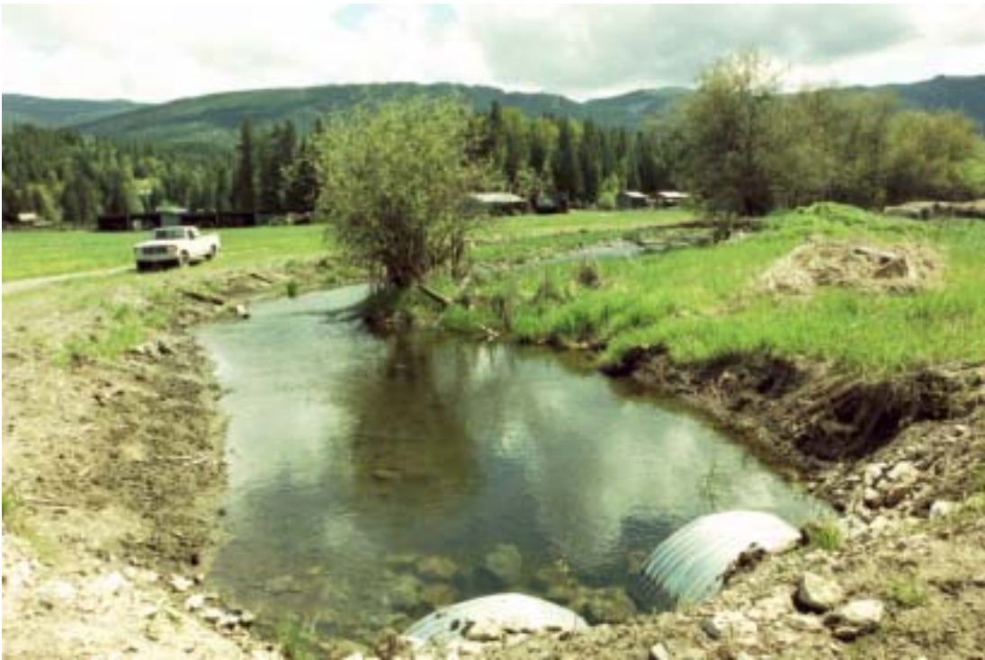
After 20: The sod was removed from the channel and the crossing upgraded.
