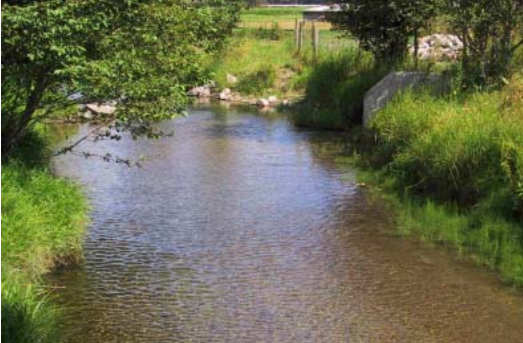
Figure 1a: Downstream view of Ireland Creek above the intake structure June 2001. The thalweg is on the left side of the stream. Sand and clumps of grass obstruct flow into the intake at low water. PP1
