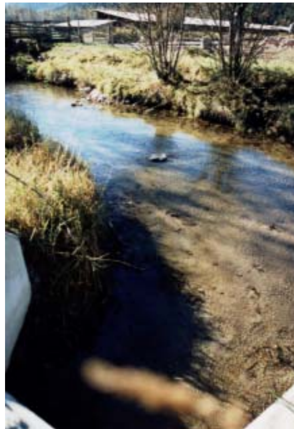
Figure 2b: The bend-away has been built, moving the thalweg toward the center of the creek. This has washed the collected sediment away from the intake. Sept 02
