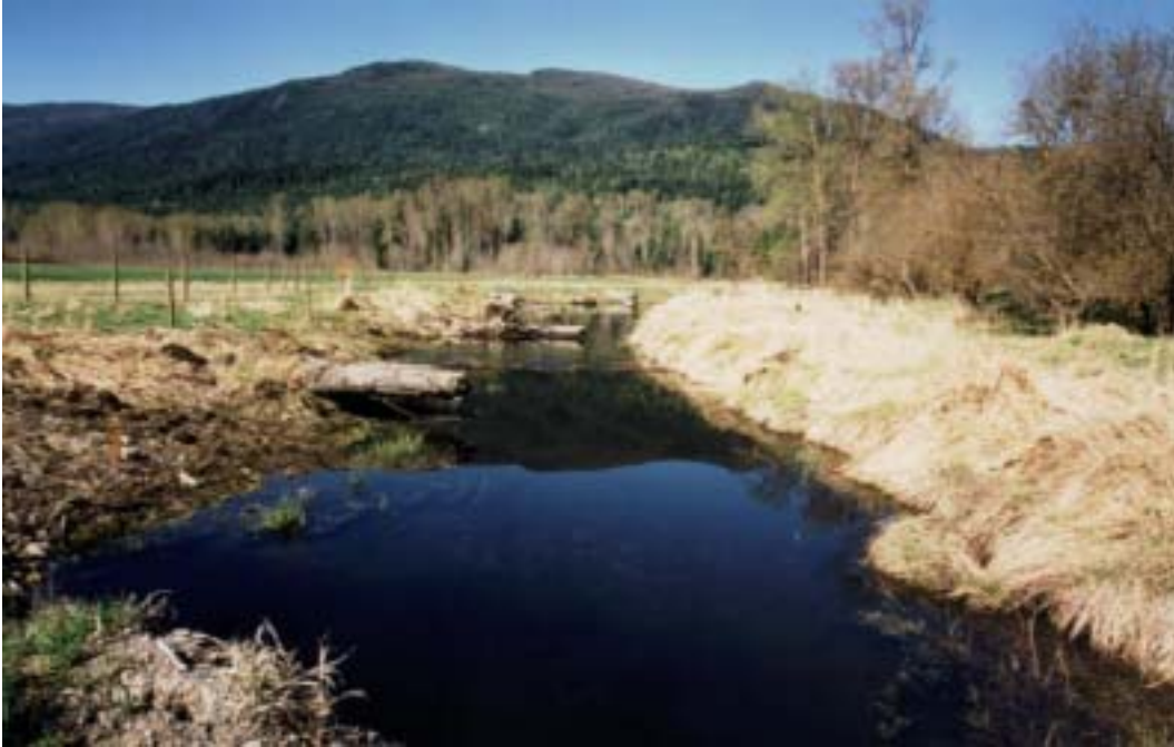
Figure 14a: 11+50 looking west before complexing. Wood had been buried into the bank during construction so that additional wood could be anchored to it.
