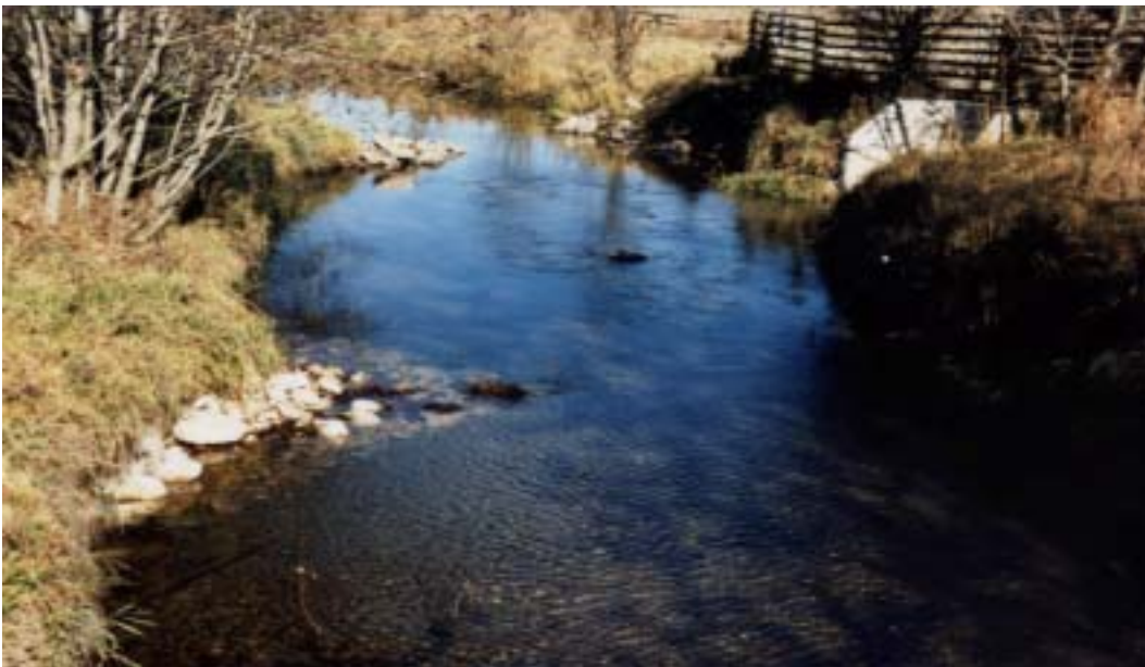
Figure 1b: A low-profile bend-away weir was built upstream of the intake to deflect the thalweg towards the intake. The sand and grass have been swept away. Sept 2002
