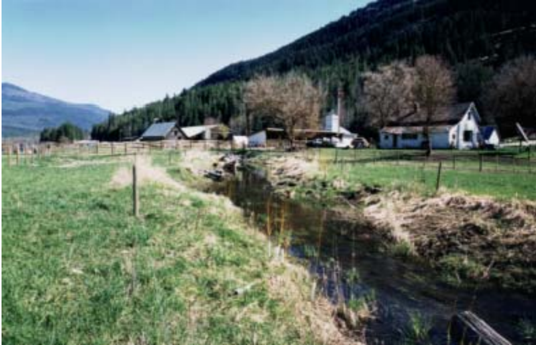
Figure 8a: 8+00 looking north before planting in May 2003
