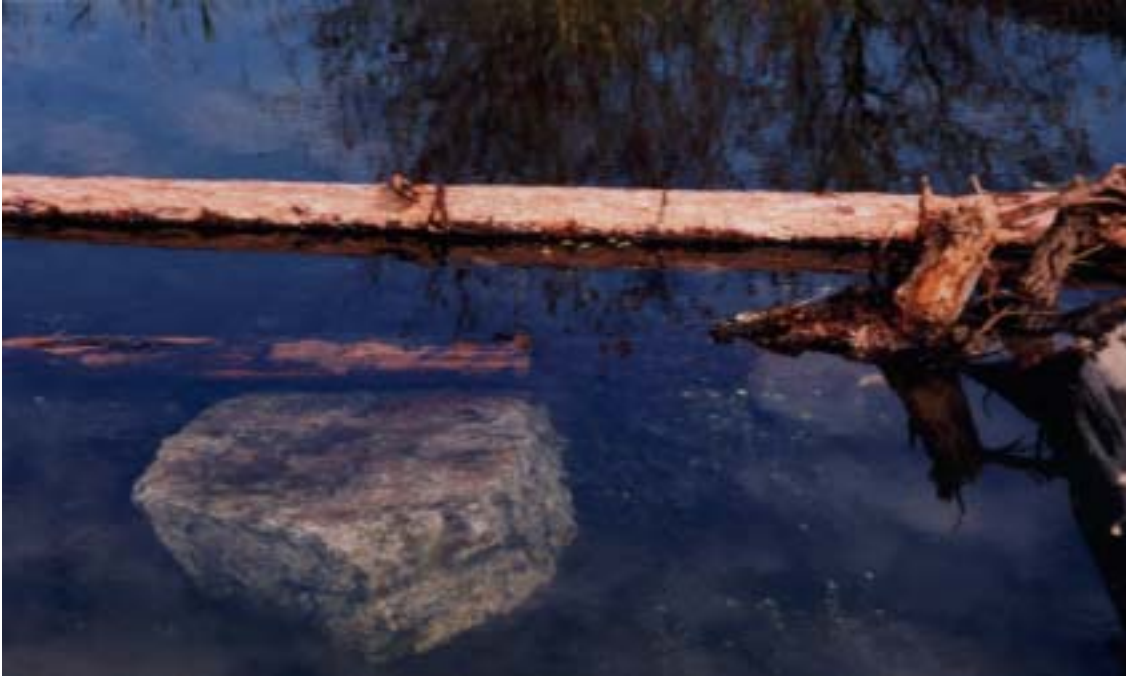
Figure 4: Chain was epoxied to holes drilled into large rocks and stapled to one or both ends of a tree. Short lengths of chain were used on approximately half the wood to provide in-stream cover. These logs are submerged even during low water. Effort was made to keep the chain hidden for aesthetic value.
