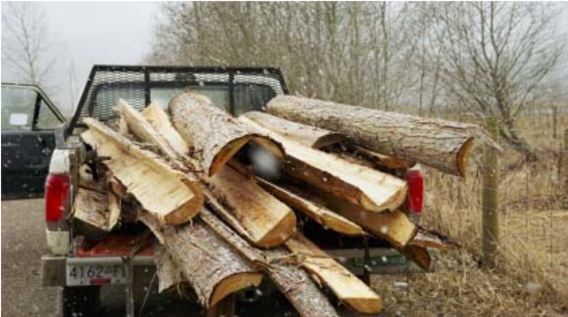
Figure 6: Cedar slabs used for complexing. The two-sided slabs are light enough to install by hand and resemble whole logs when placed in the water. The cavity provides more in-stream cover than whole logs.
