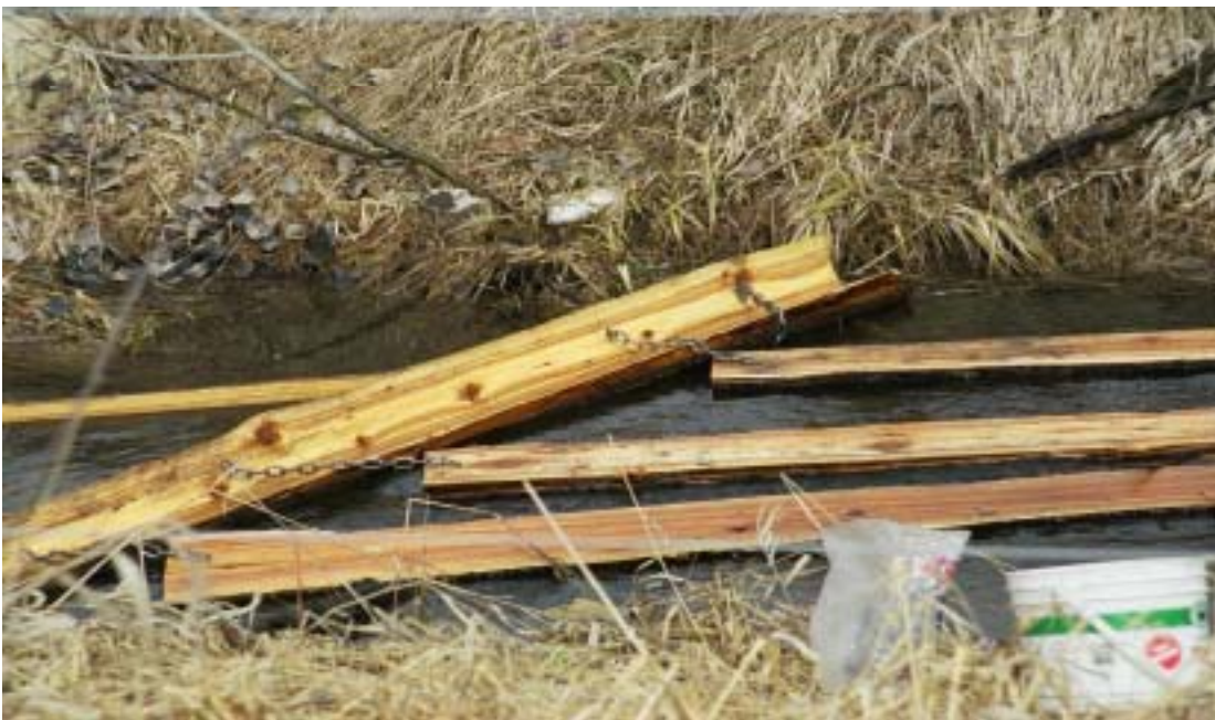
Figure 7: The slabs can be chained underneath so the chain is not visible.
