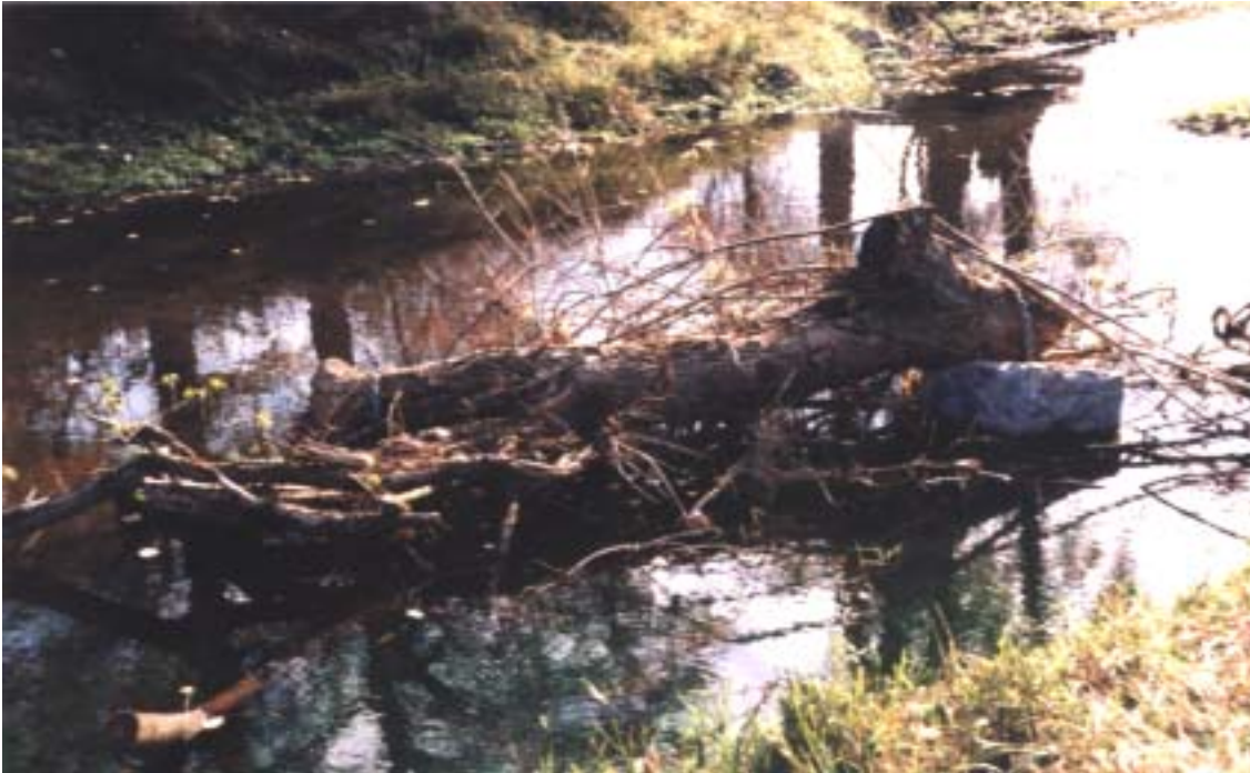
Figure 5: Brush was piled in pool areas and held in place by logs placed on top of the pile. The logs were anchored weighted with rock.
