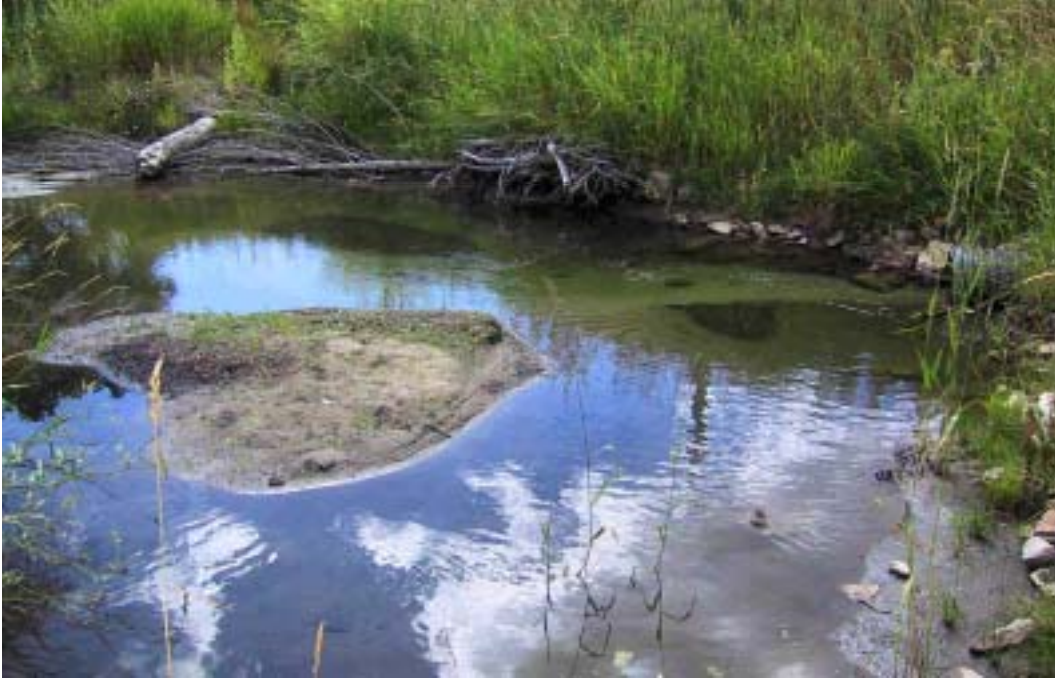
Figure 13: Sediment has filled the collection pond at the intake structure. June 01
