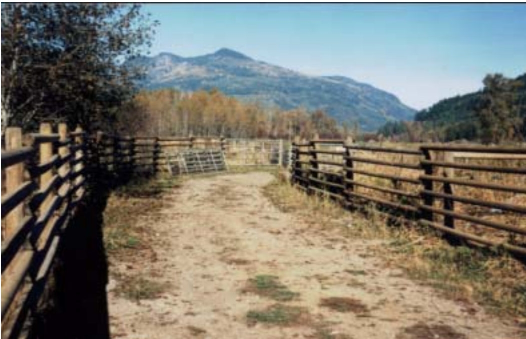
Figure 17: Rails were placed at the uppermost crossing where hogs are frequently moved. The bottleneck pressure was too much strain on just the page wire fence.
