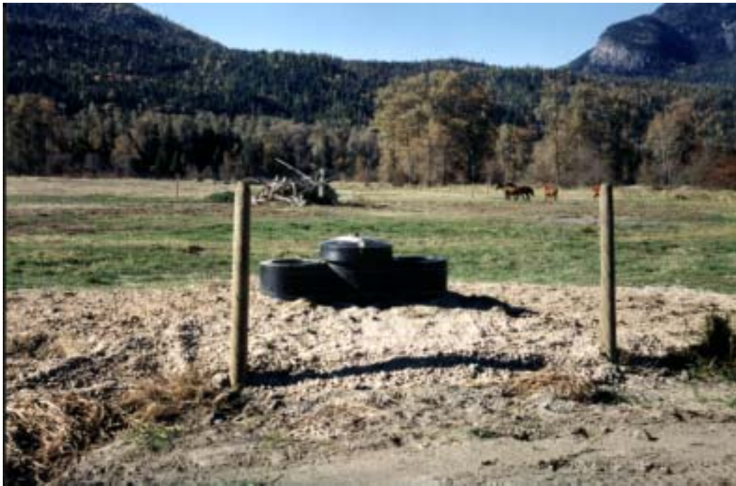
Figure 15: The waterer was installed outside the fenced riparian area. The tank is largely underground and the above ground part of the structure is insulated. The water stays ice-
