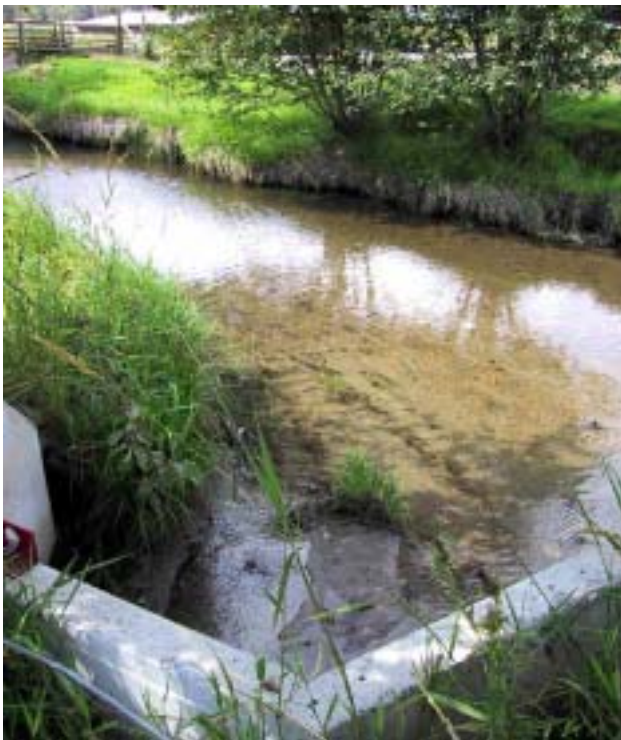
Figure 10: A low profile bend-away upstream of the intake kicks the thalweg to the right bank. The rocks located downstream were in place prior to construction.
