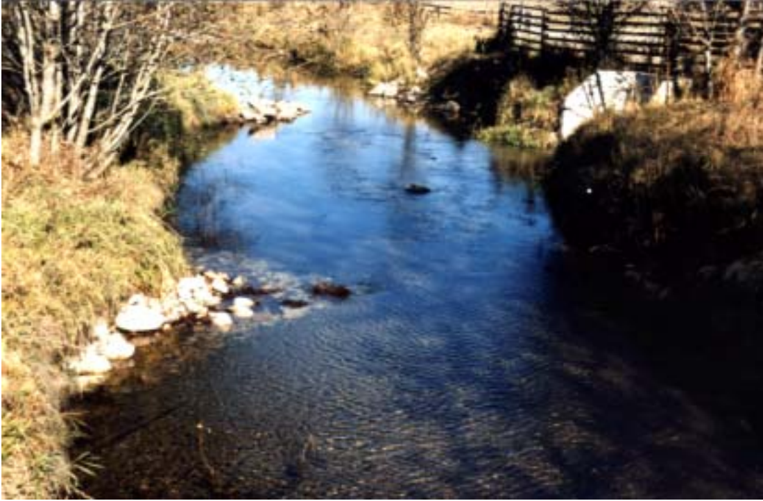
Figure 10: A low profile bend-away upstream of the intake kicks the thalweg to the right bank. The rocks located downstream were in place prior to construction.
