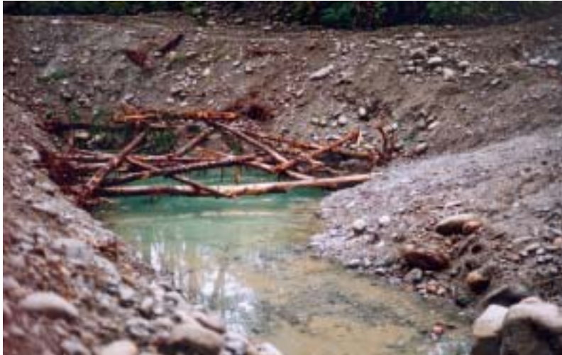
Figure 9. Upstream end of the groundwater channel before the final grading of the channel.
