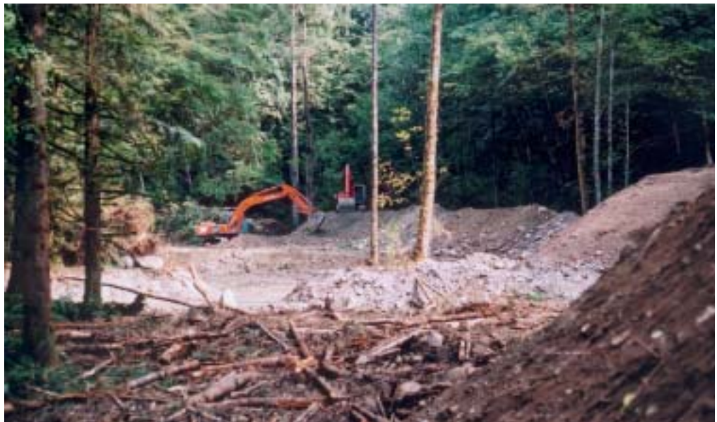
Figure 7. Looking east- northeast to the north half of the north pond. Machines are spoiling the shallow pass gravel onto a separator berm to protect the habitat from the Unnamed Creek to which it drains.
