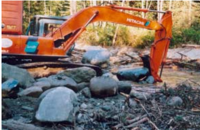
Figure 5. South pond during deepening work
