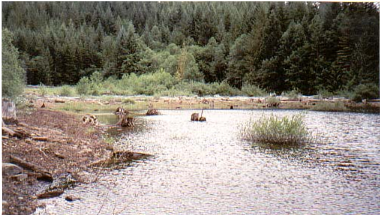
View to southeast end of Elsie dam and track plate 12
