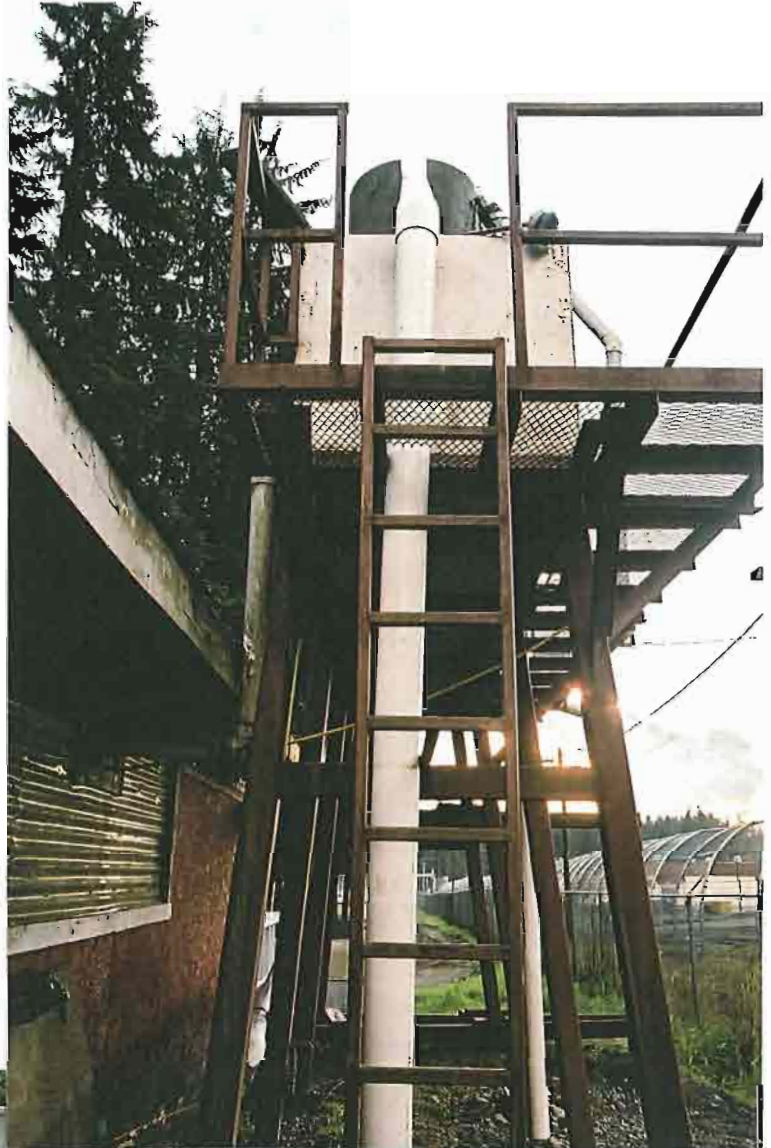
Photo 9: Allco springs discharge pipe in aeration tank above upper hatchery.
