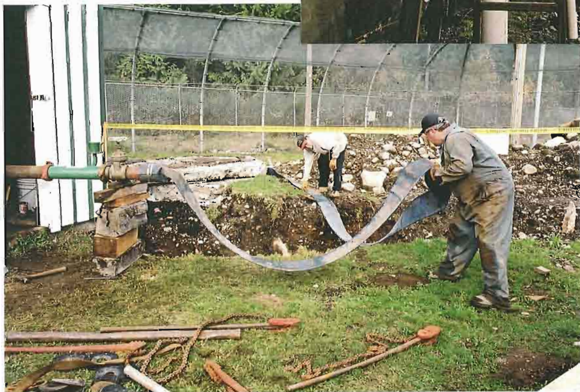
Photo 10: Flat hose being laid for well pump performance test.
