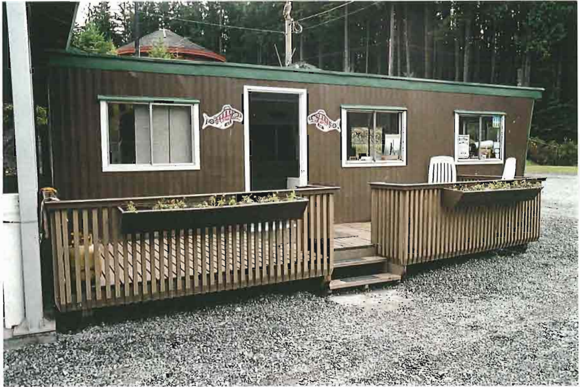
Photo 13: Allco's new hatchery office illustrating another FOC, Allco Hatchery, ARMS partnership.
