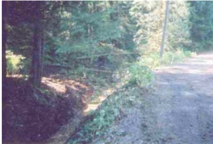
Figure 1. Channel along east side of Alouette Dam road (looking south).
