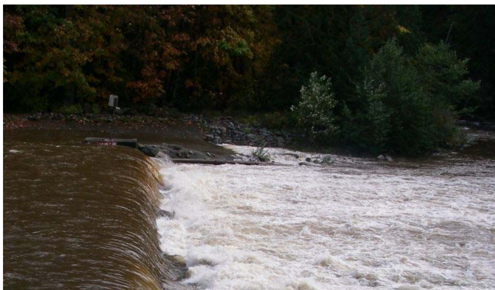
Photo 3. Barrier fence in the Puntledge River at the Lower Hatchery showing the bypass channel created on the left bank, accessible by summer chinook during freshet flows. Photo taken during a discharge of 77 cms (measured at Gauge 8).
