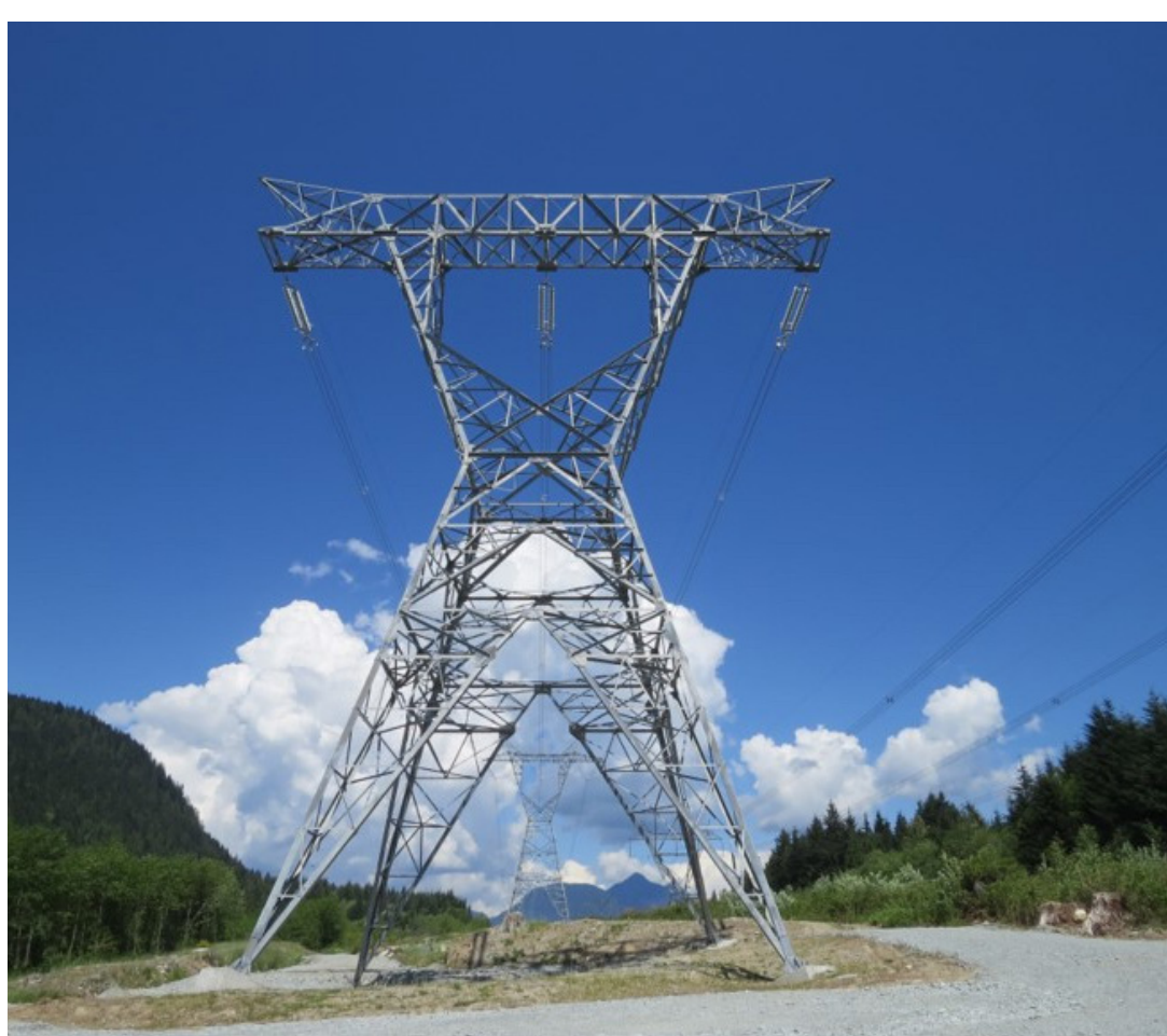
500kV Self Support Lattice Dead-End
