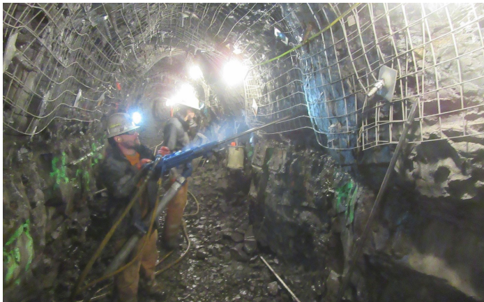
Refurbishing the existing rock support elements at the Peace Canyon left adit – a passage located in the dam abutment.
