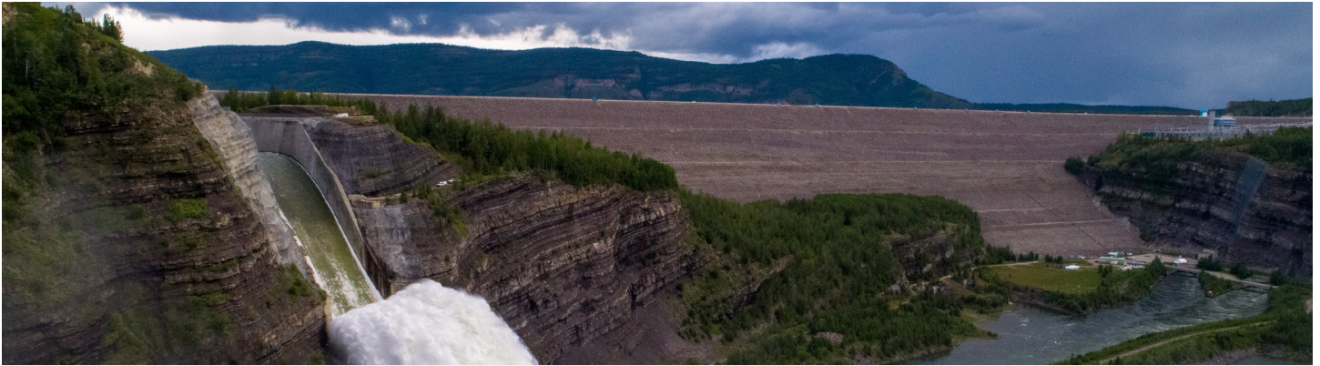
The W.A.C. Bennett Dam spillway was in use for short periods during the last two summers including this spill during July 2020.
