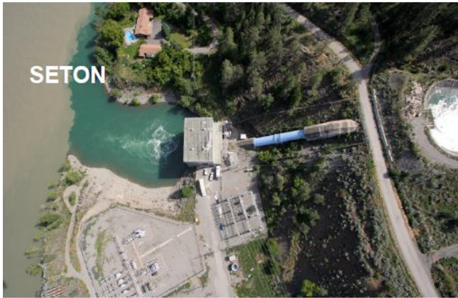
Aerial view of the Seton penstock and generating station
