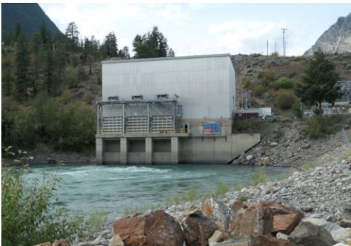
Above: Seton Dam. Below: Seton Powerhouse
