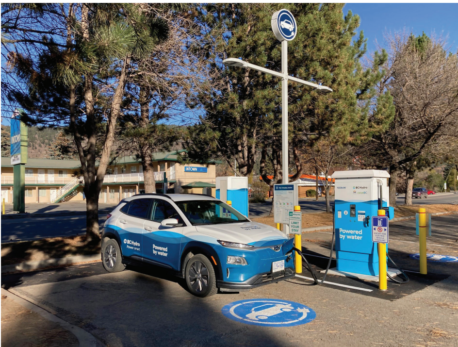
Figure 2: Example of a BC Hydro light pole assembly
