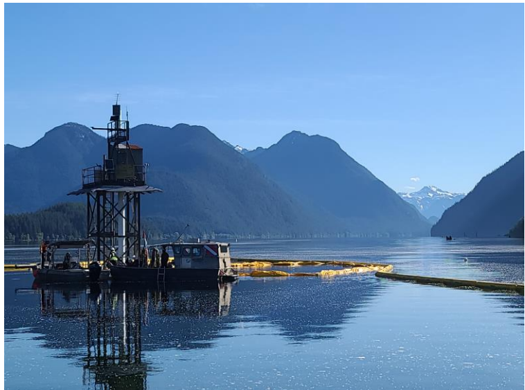
Figure 5 Alouette Dam low level intake with dredging underway.
