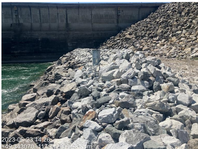
Figure 8 Hugh Keenleyside completed tailrace north bank modification. A berm has been constructed in front of the flat bench to prevent fish stranding.
