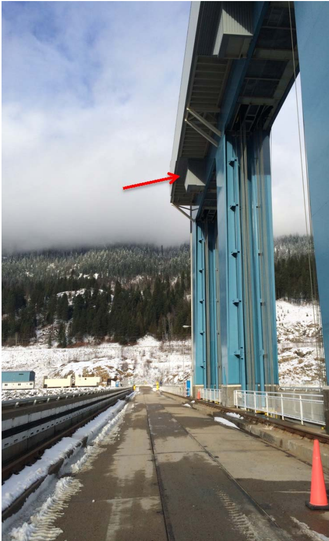
Hatch located directly above dam deck.
