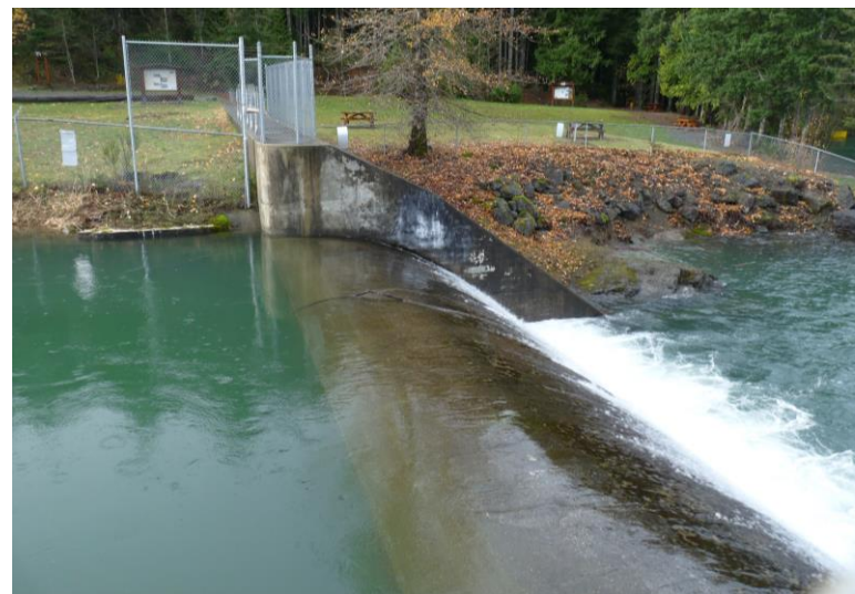
Photo 3 – Spilling over the Free Overflow Spillway
