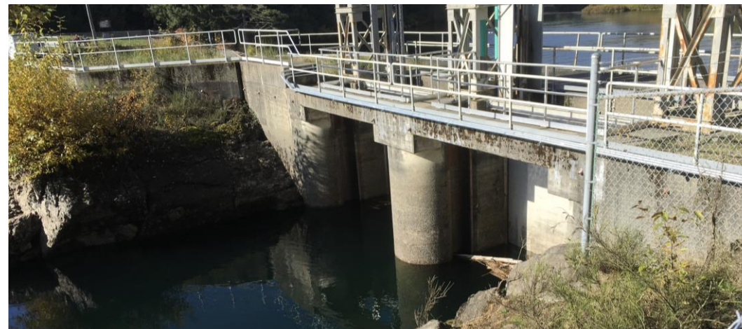
Photo 5 – The upstream side of the Sluiceway at low flow
