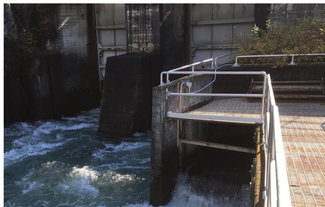
Photo 4 – Downstream face of Sluice Gates and Fishway
