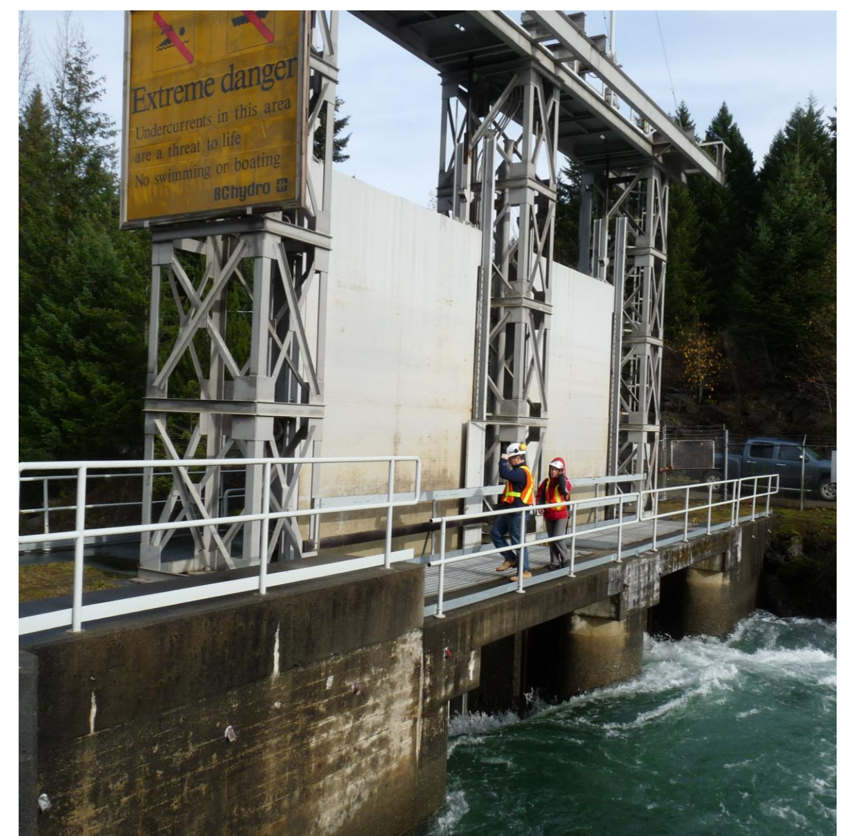
Photo 6 – Passing flows with Sluiceway gates fully open
