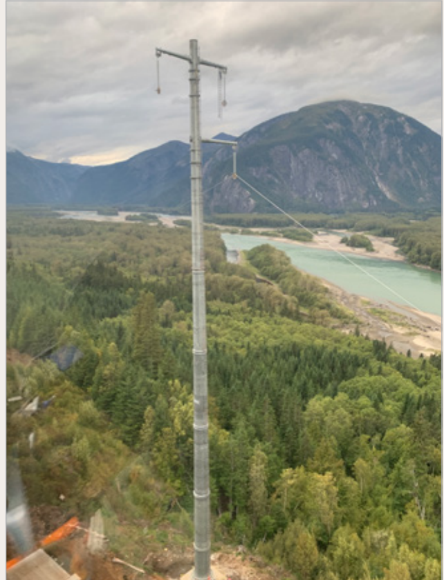
Figure 15: One of the new poles in place
