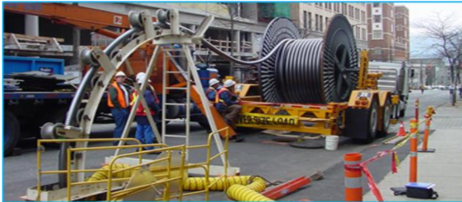
An example of placing cable.
