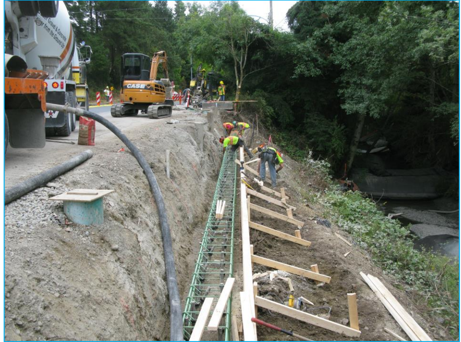
Photos from 2013: Soil remediation work to remove mineral oil beside Colquitz Creek. The work also included bank stabilization
