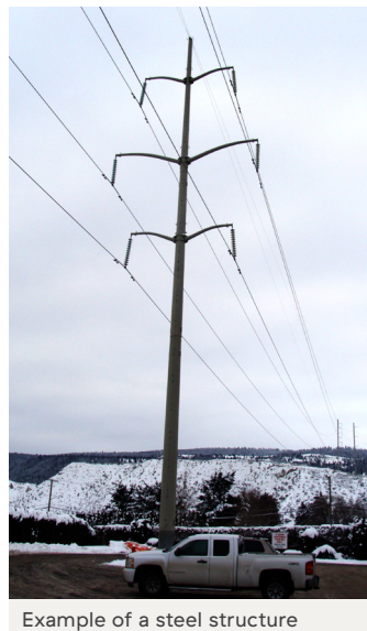
Example of a steel structure
