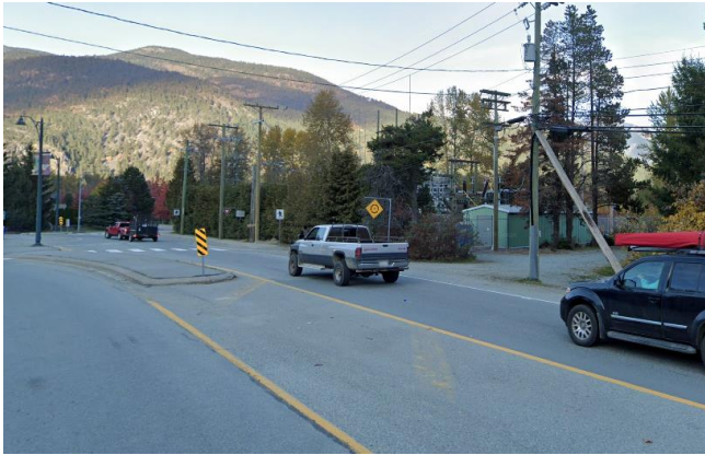
View from Pemberton Portage Road near Portage Road, looking north. Substation is to the right.
