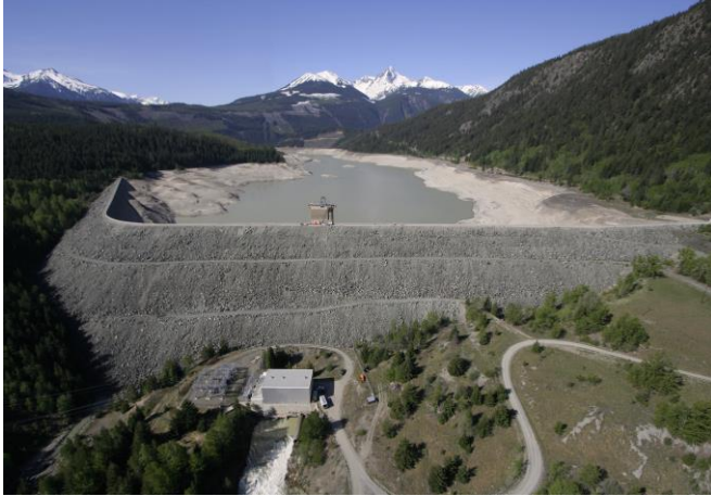
LaJoie Dam with Downton Reservoir in the background and a 25 MW powerhouse in the foreground
