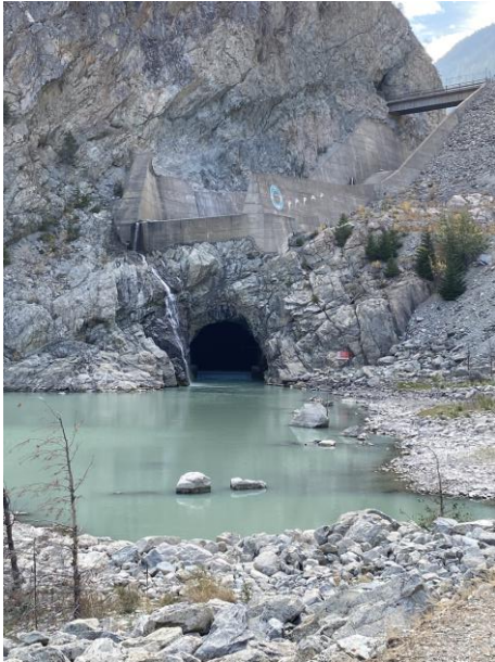
Terzaghi spillway and low-level discharge outlet
