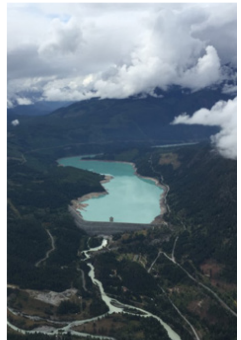
Aerial Shot of LaJoie Dam and Generating Station with Downton Reservoir.
