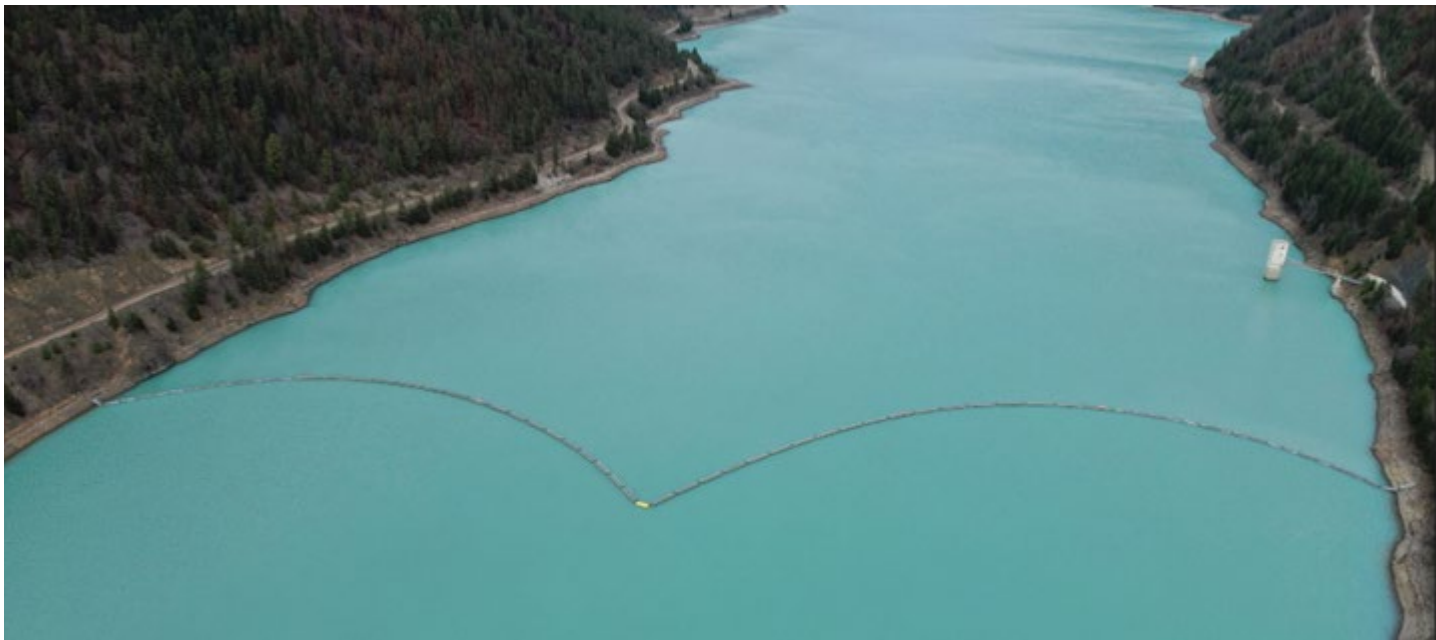
Figure 10 The new reservoir boom on Carpenter Lake. The intake structures for Bridge River 2 (at front) and Bridge River 1 (at back) are visible on the right side of the reservoir. Terzaghi Dam is just beyond the top of the photograph.
