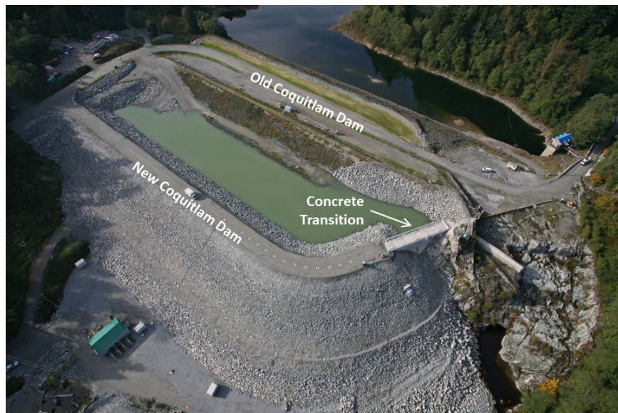
Figure 6 Above: Coquitlam Dam and the concrete transition structure. Right: Setting up the equipment to pull-test the concrete transition's three post-tensioned anchors.
