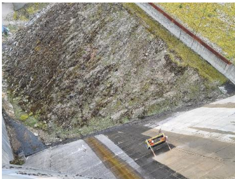
Figure 5 Workers pressure washing the Revelstoke Dam Transition Blocks.
