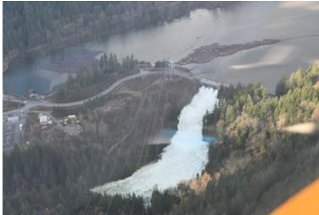
(a) November 16, 2021 spill of approximately 1500 cubic metres per second (near the event's maximum spill) at Stave Falls (Blind Slough Dam).
