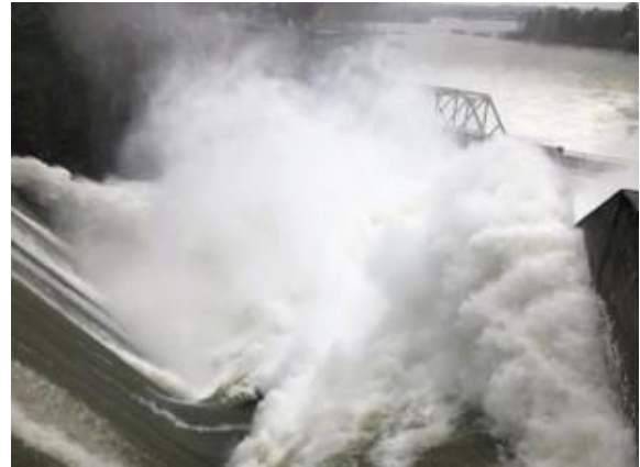
(b) November 15, 2021 spill of approximately 1300 cubic metres per second (near the event's maximum spill) at Ruskin Dam.
