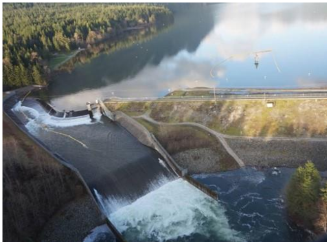
(c) December 2, 2021 spill of approximately 70 cubic metres per second (about 80% of the event's maximum spill) at Alouette Dam.
