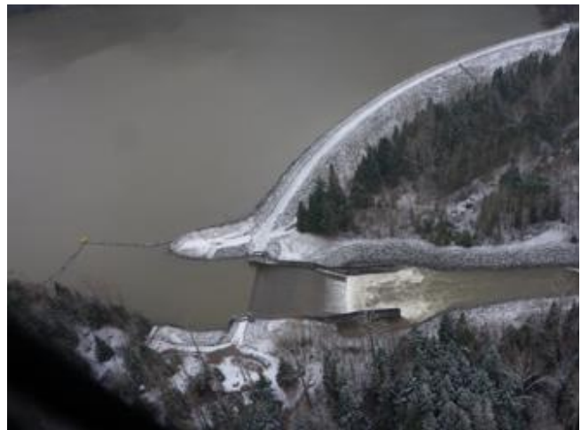
(d) November 16, 2021 spill of approximately 50 cubic metres per second (about 50% of the event's maximum spill) at Wahleach Dam.
