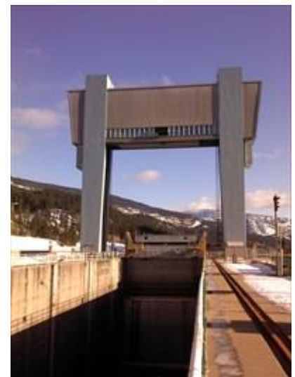
Figure 4 Downstream gate and control/hoist tower of the Hugh Keenleyside Dam navigation lock.
