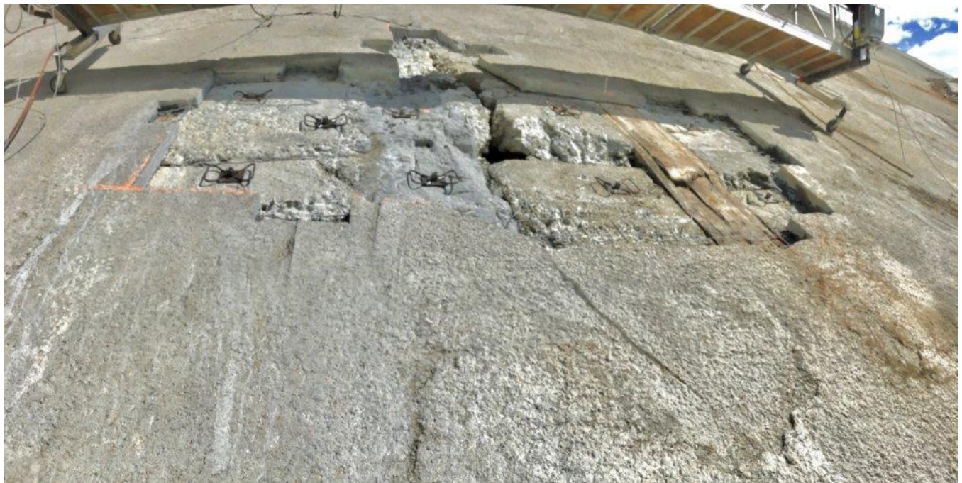
Figure 5 Shotcrete undergoing repairs on the La Joie dam face.
