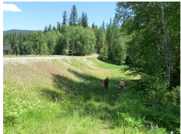
Downstream face of the Saddle Dam
