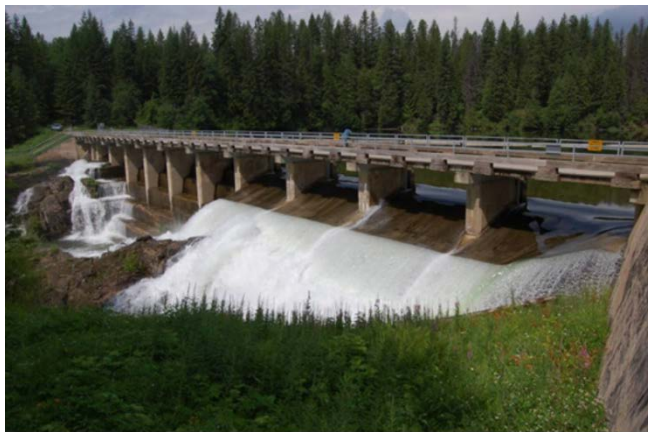
Whatshan Dam – Spillway in operation
