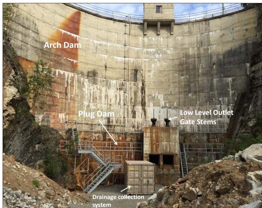
Wilsey Dam view from the downstream following F2016 work
