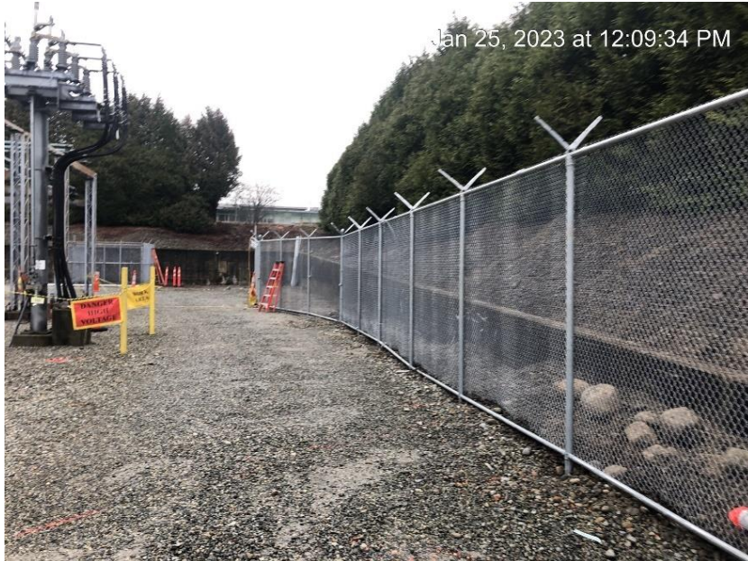
Figure B-1 Temporary 2.4-meter-high metallic fence installed on south side of the property, January 2023
