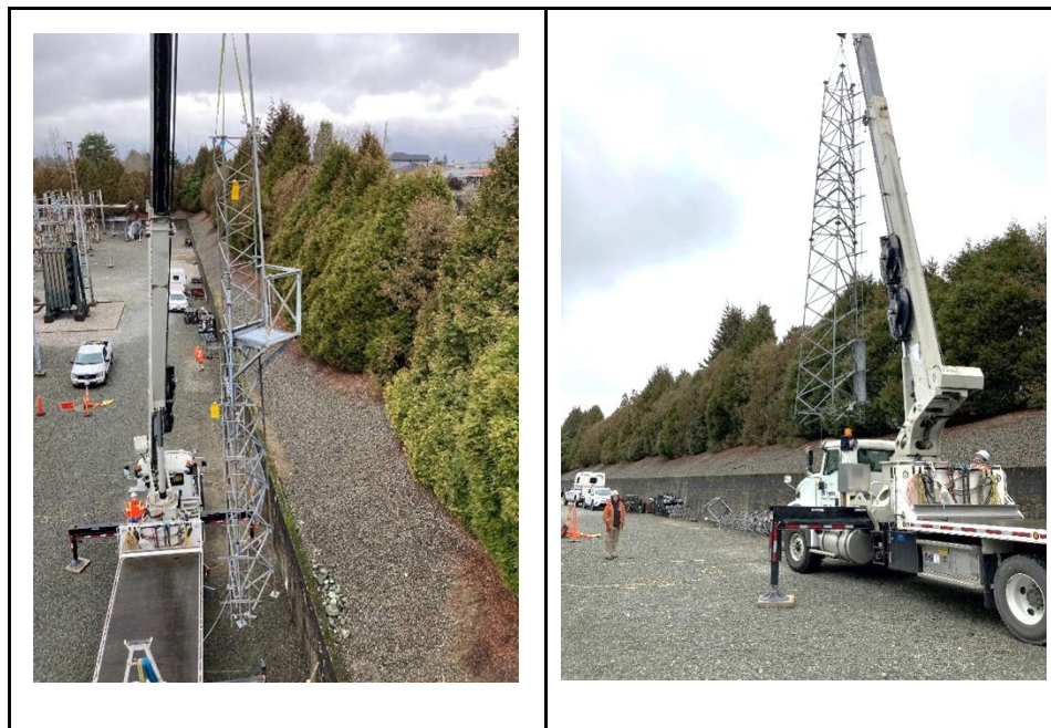
Figure B-6 Removal of the existing microwave tower, southeast corner of substation, February 2023
