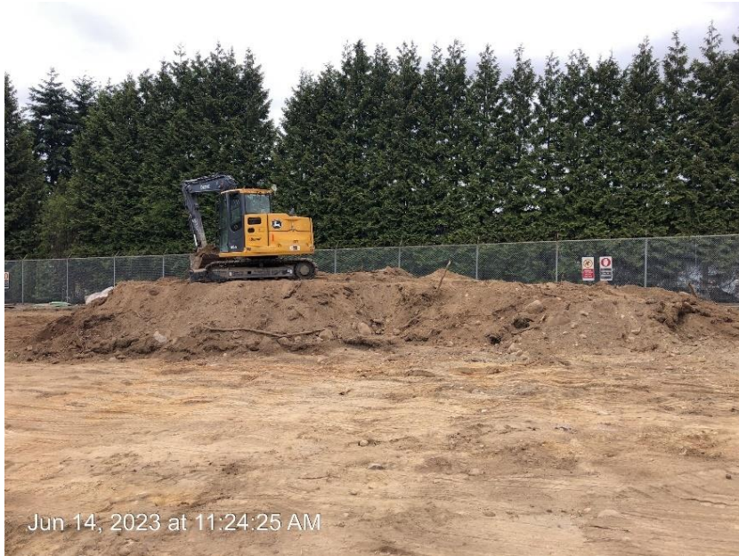
Figure B-7 Excavation of soil for the new gas insulated switchgear feeder building on the south-west side of the substation property, June 2023
