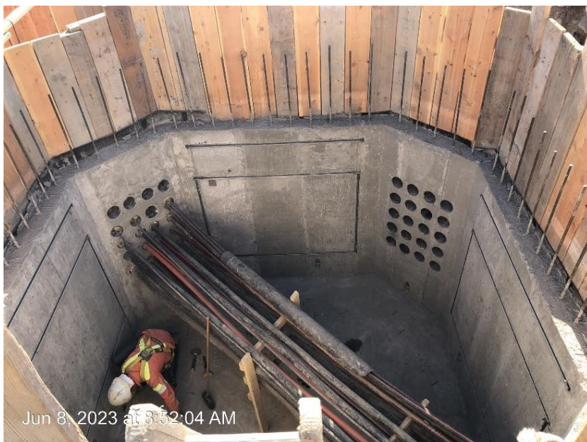
Figure B-8 Installation of new four way distribution maintenance hole, June 2023
