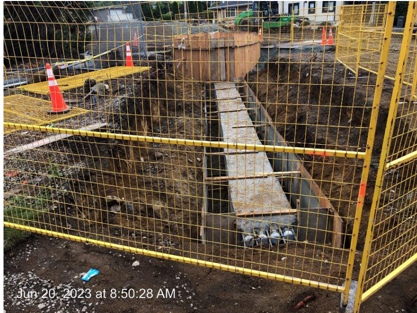
Figure B-9 Installation of new distribution duct bank, June 2023
