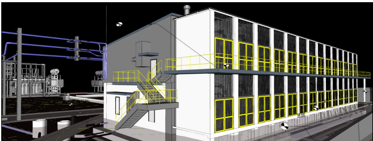
Figure A-2 Rendering of gas insulated switchgear feeder building design showing building exterior
