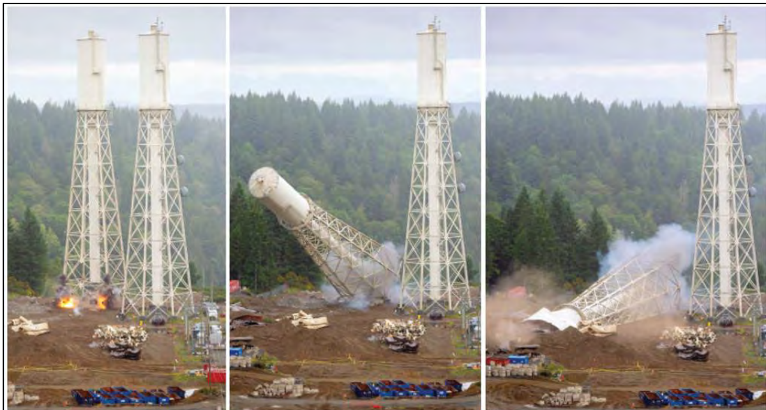
Figure A-13 Second Surge Tower Removed
