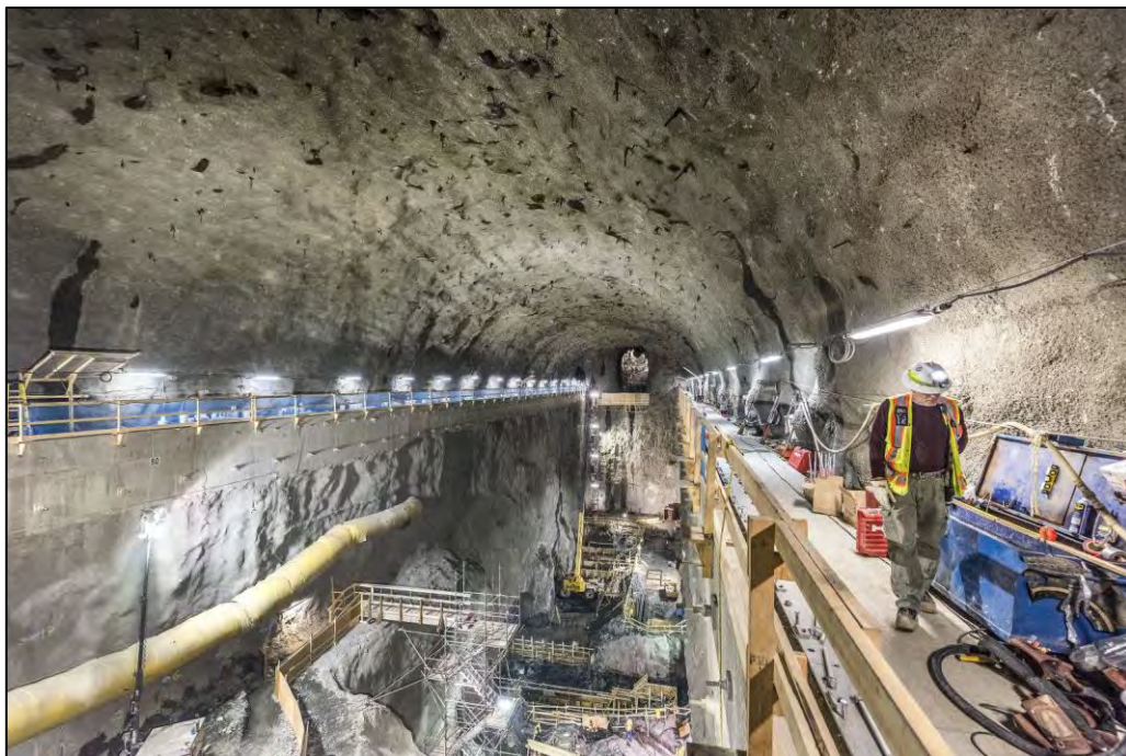
Figure A-23 Powerhouse Cavern (August 2016)
