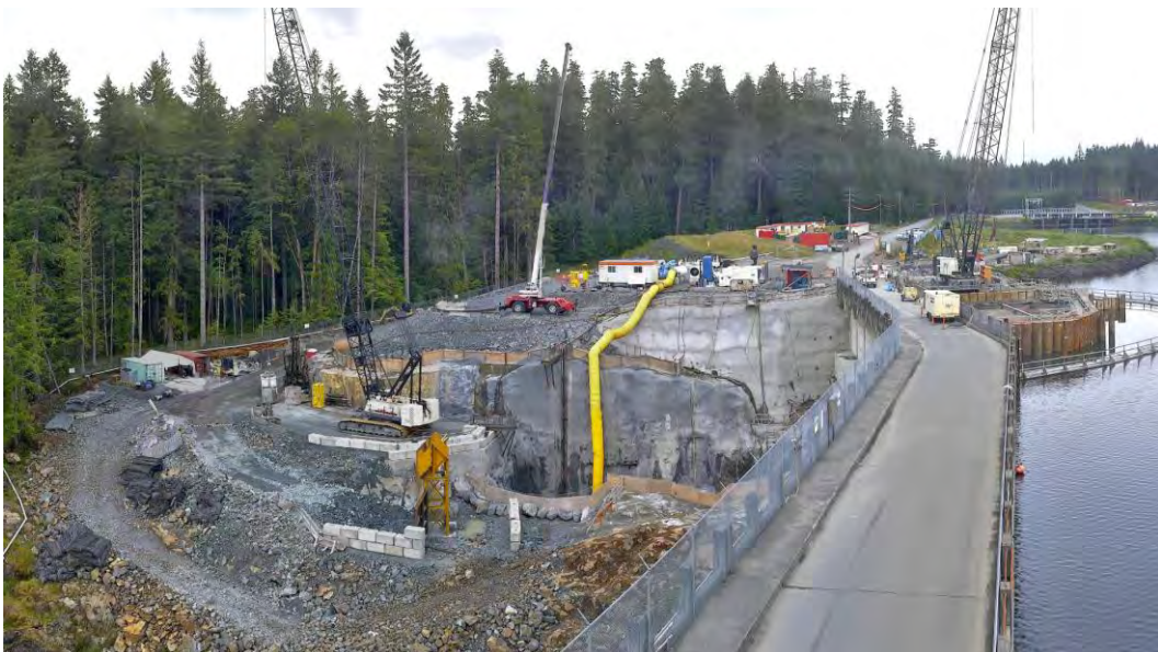
Figure A-6 June 2016 - Intake Drop Shaft Excavated
