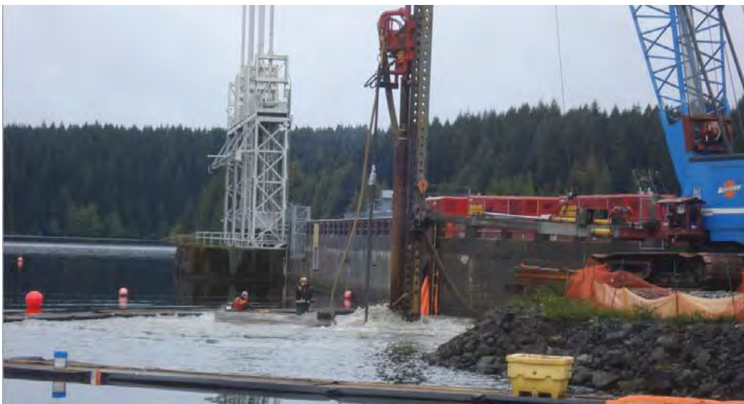
Figure A-4 April 2015 Cofferdam Pile Installation
