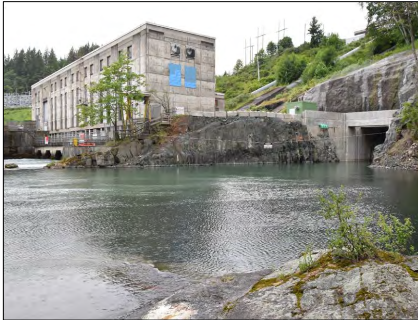
Figure A-16 Old Powerhouse
