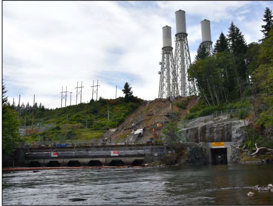
Figure A-18 Old Powerhouse Removed
