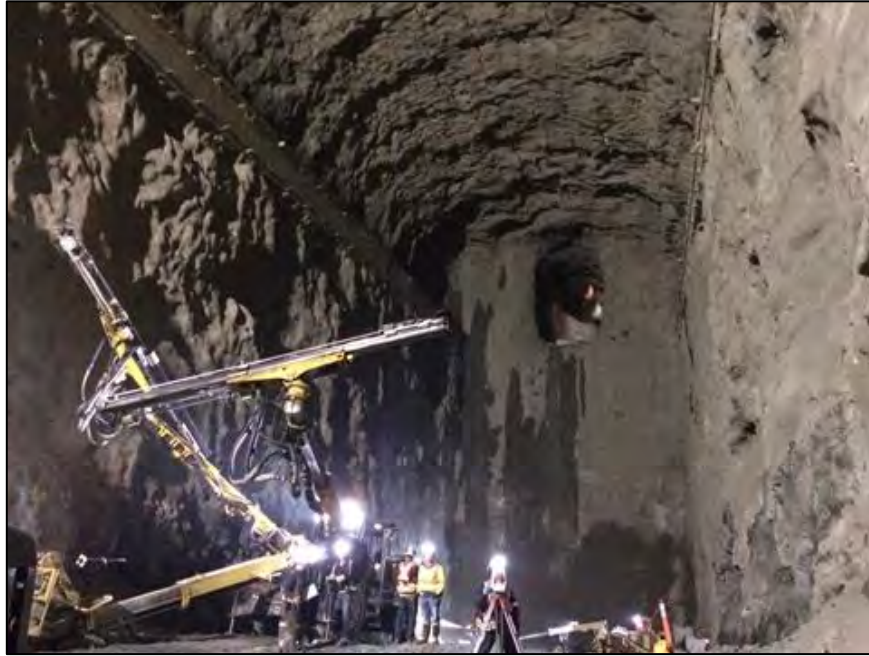
Figure A-22 Powerhouse Cavern (April 2016)
