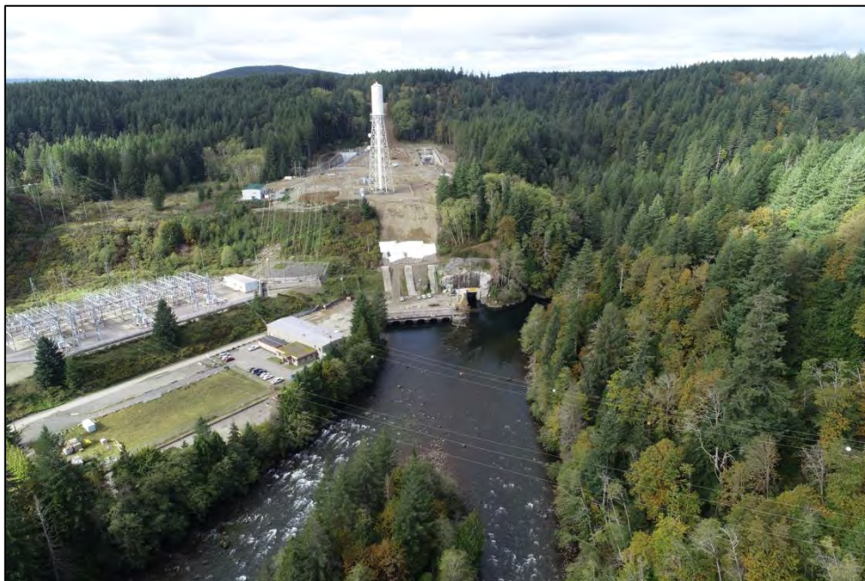
Figure A-9 Powerhouse and Surge towers removed
