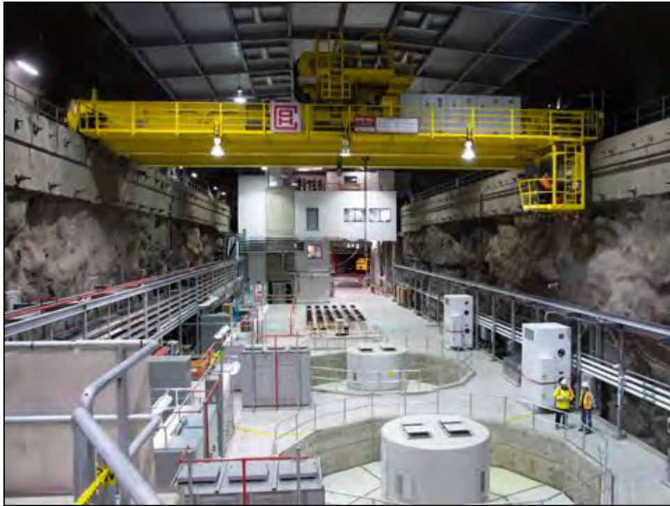
Figure A-24 Powerhouse Cavern (December 2018)
