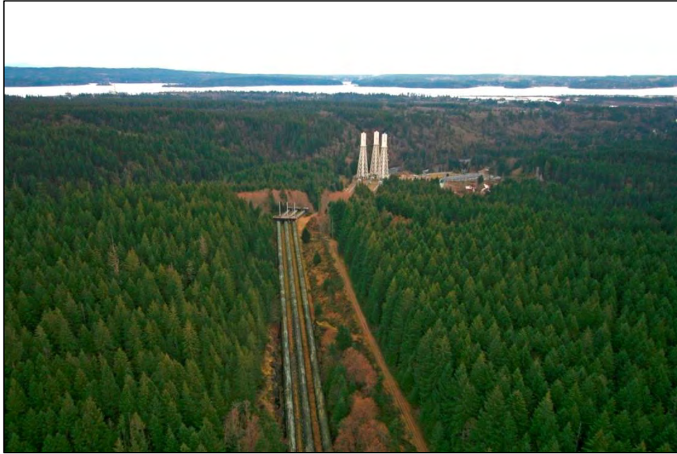
Figure A-14 Penstocks
