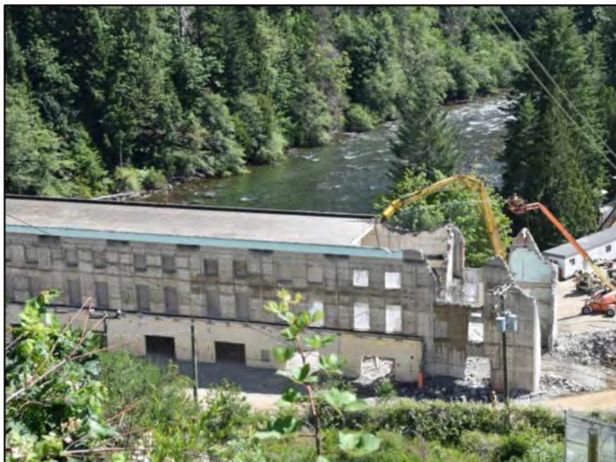
Figure A-17 Powerhouse Demolition
