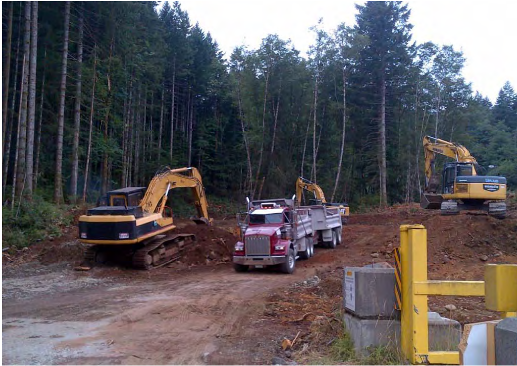
Figure A-1 Clearing Work at South Portal (07/14)
