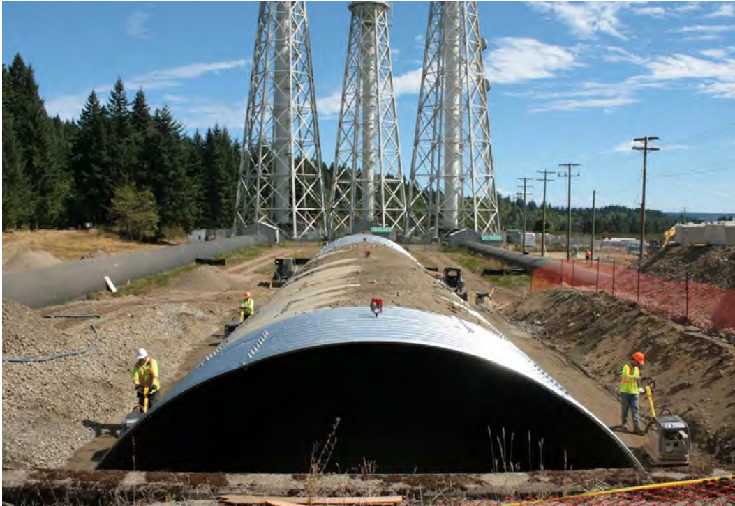
Figure A-3 Building Temporary Penstock Crossing to North Portal (08/14)
