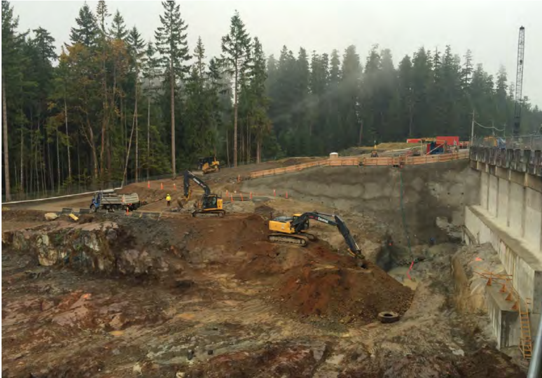
Figure A-5 September 2015 Excavation downstream of Dam
