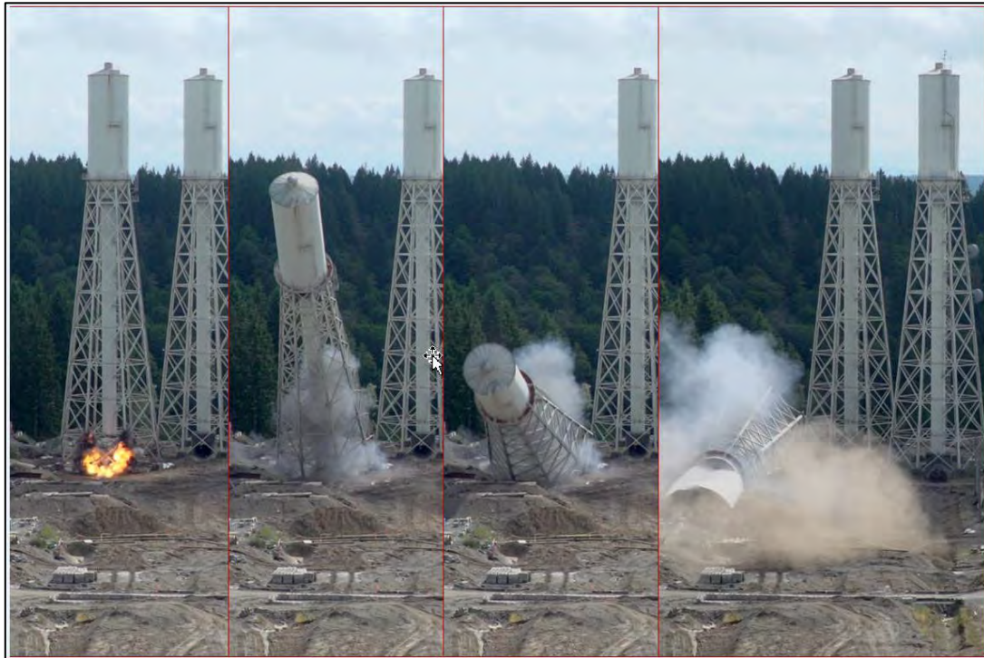
Figure A-12 First Surge Tower Removed
