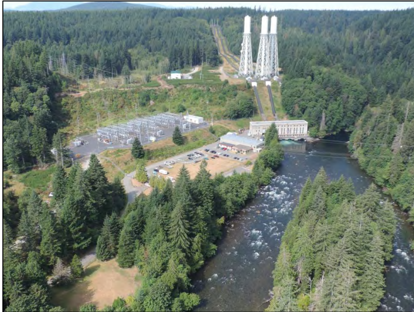
Figure A-8 Existing Powerhouse and surge towers before removal
