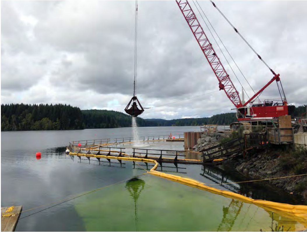
Figure A-7 Oct 2017 Removing Blasted Rock from Intake Channel
