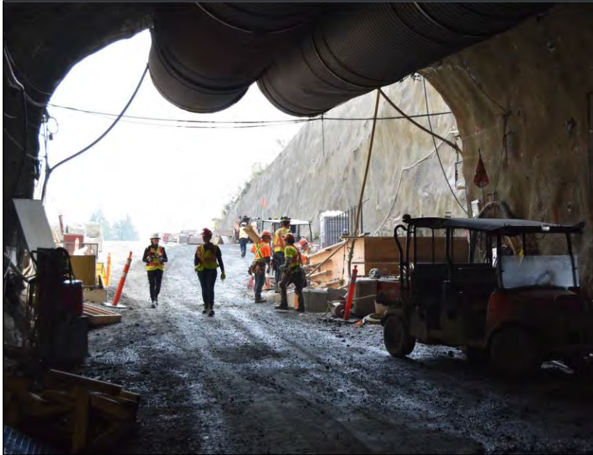
Figure A-20 Main Access Tunnel North Portal
