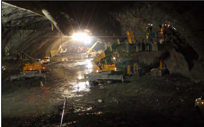
PHOTO 9 – Ingula Pumped Storage Scheme – Machine Hall Under Construction.
