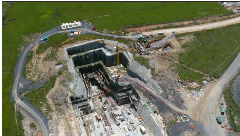
PHOTO 10 – Ingula Pumped Storage Scheme – Outlet Structure Under Construction.
