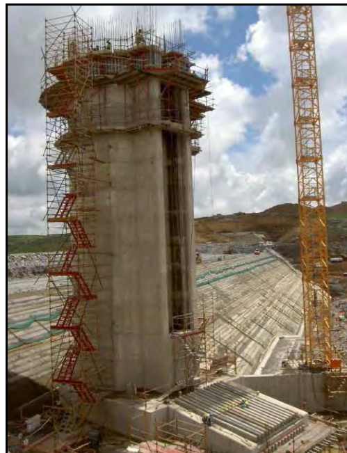
PHOTO 8 – Ingula Pumped Storage Scheme – Intake Tower Under Construction.
