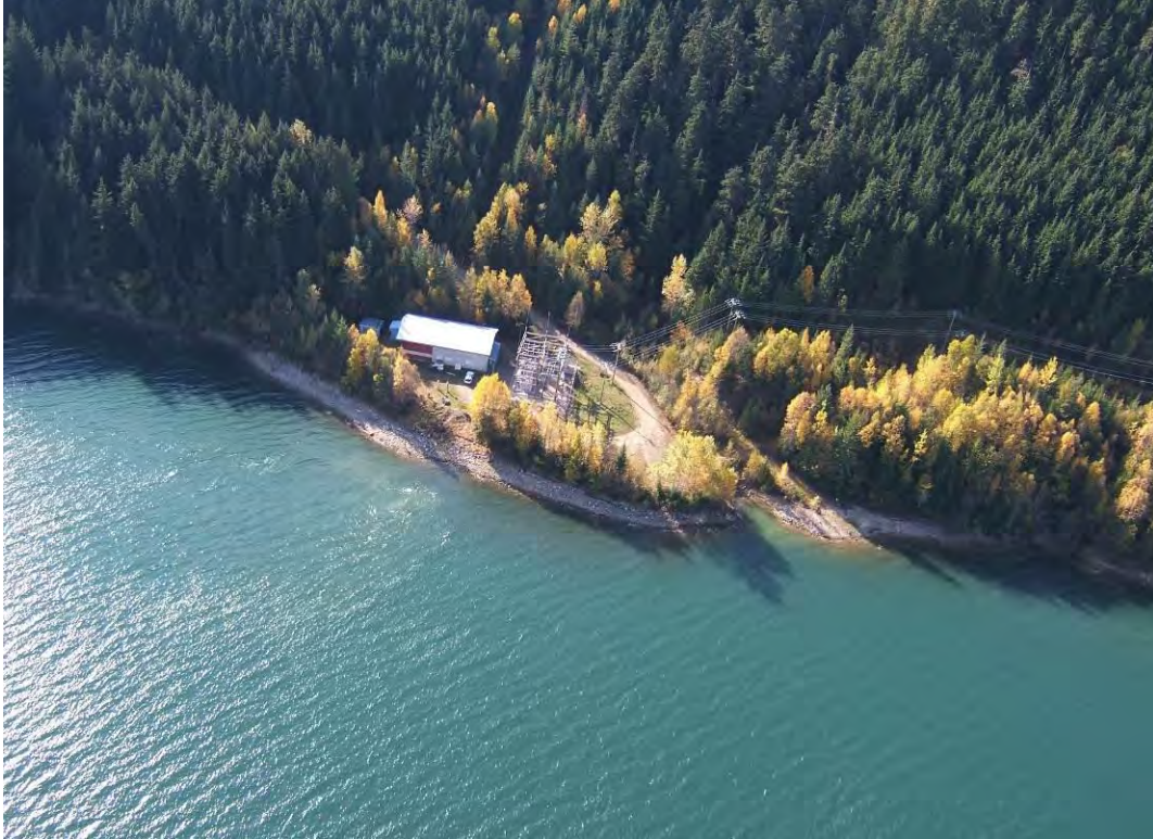
Walter Hardman Generating Station located on the west shore of Arrow Lakes Reservoir (October 10, 2008, ALR elevation 437.95m)
