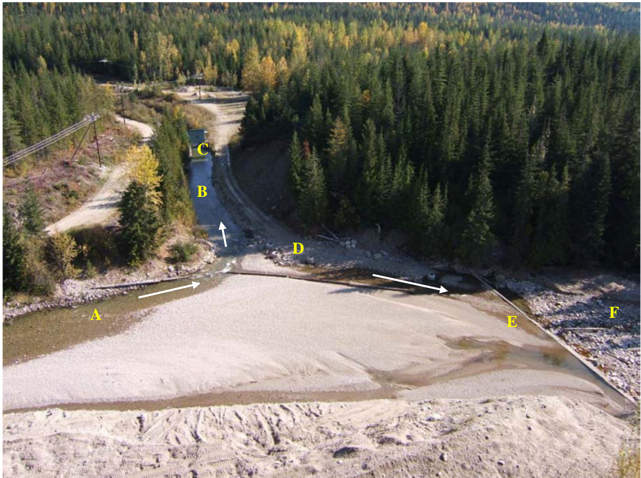
Figure 1-2. Overview of the minimum flow release facility at Walter Hardman, looking east (Sept 18 2008). (A) Upper Cranberry Creek, (B) Diversion channel, (C) Headworks Operating Gate, (D) Drywells (intakes), (E) Diversion Dam, (F) Upstream end of lower Cranberry Creek. (BC Hydro 2009)
