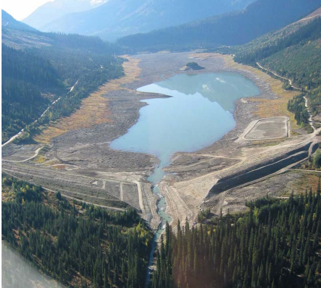
Photo 2-1: Coursier Dam Decommissioned. A notched channel was cut through the dam structure, and the lake is returning to a natural cycle (October 2003 picture).
