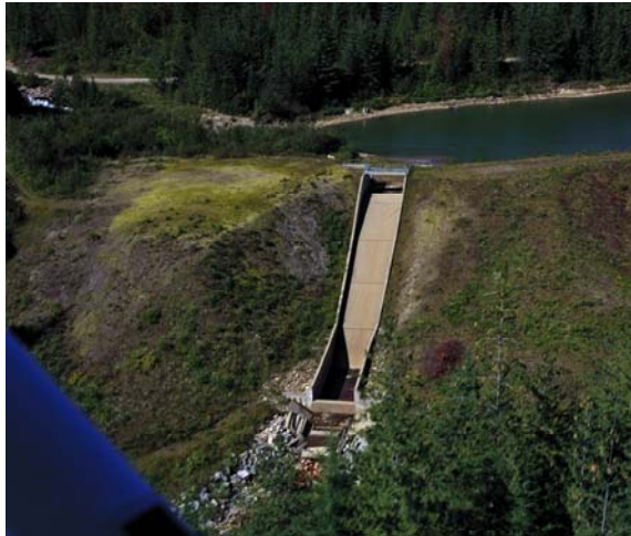
Photo 2-6: Spillway on Cut-off Dam at Walter Hardman Headpond
