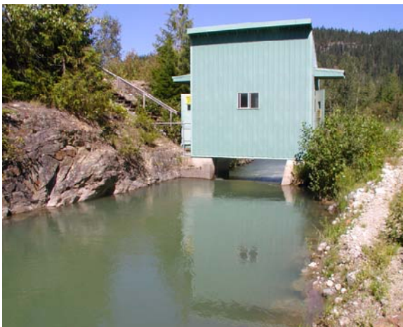
Photo 2-3: Stoplog Control Structure (left, facing downstream in diversion channel)
