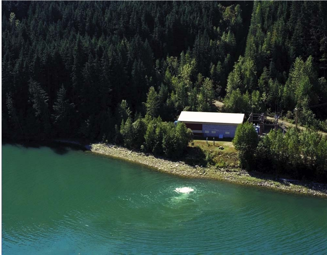
Photo 2-8: Walter Hardman Generating Station on Upper Arrow Lakes Reservoir
