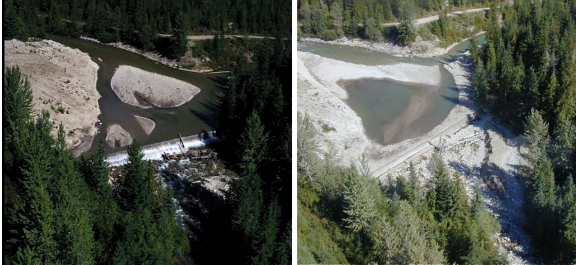
Photo 2-2: Diversion Dam, with Freecrest Overflow (left) and No Overflow (right)
