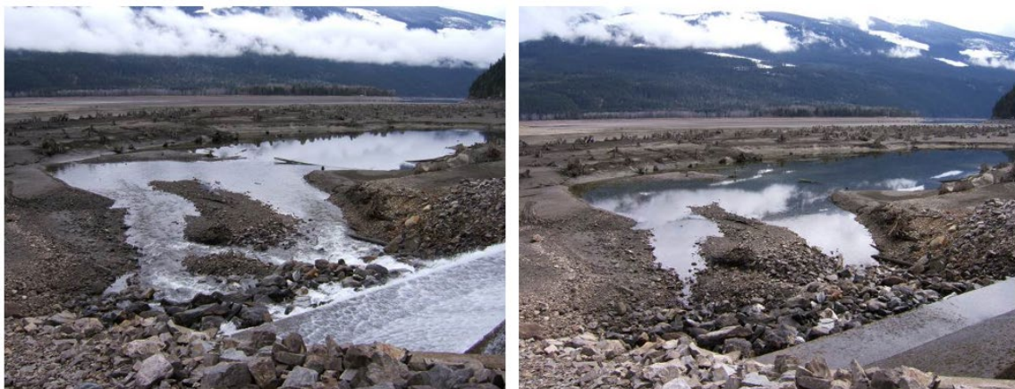
Figure 5.6.b: WHN powerplant outlet structure and back channel, before and after plant outage, April 17, 2012.
