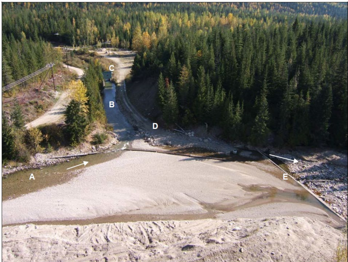
Figure 4.1.b Overview of the minimum flow facility looking east (Sept. 18, 2008). (A) Cranberry Creek, (B) Diversion channel, (C) HWOG (replaced former stoplog structure), (D) Drywells (intakes), (E) Diversion dam and arrow indicating minimum flow outlet.
