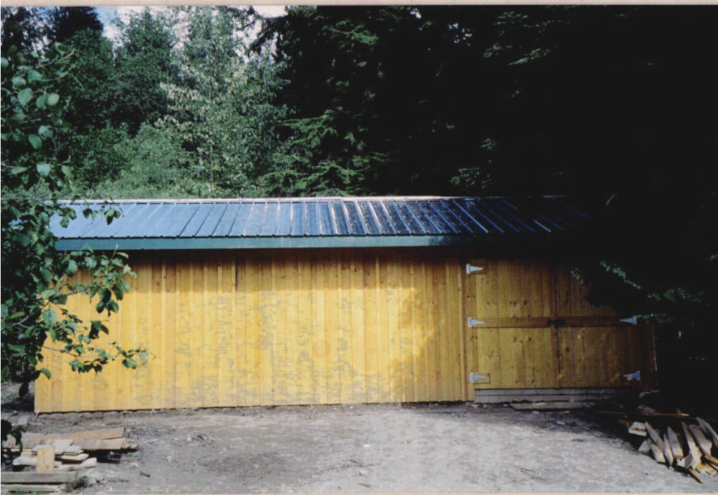
Photo 2. New tank farm constructed in 2006. Facility is a cedar shed with a metal roof to withstand heavy snow loads and a locking door.
