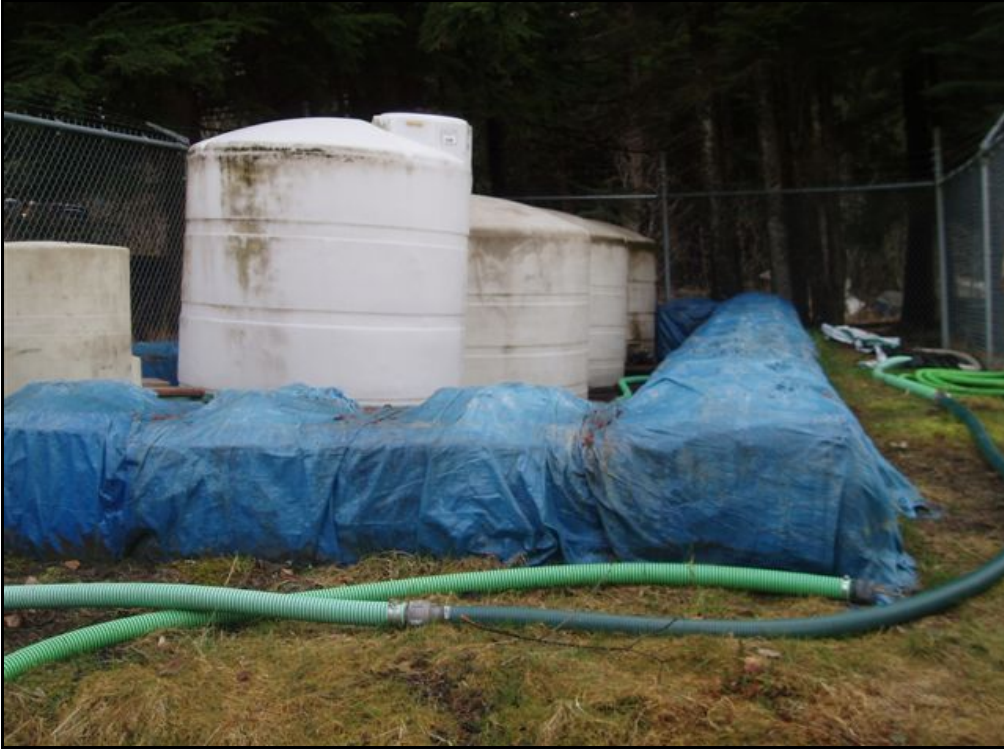
Photo 1. Old tank farm, consisting of a concrete berm covered with a tarp, and chain link fence.
