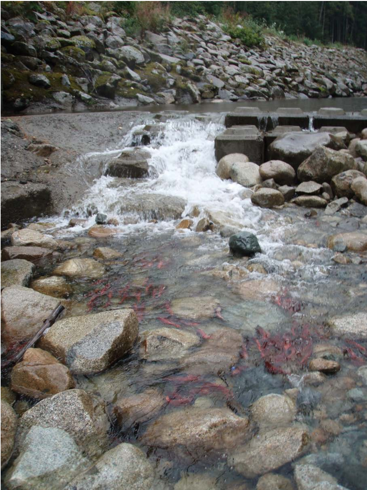
Photo 3. Upgraded weir on Boulder Creek blocking access to spawning ground, September, 2006.
