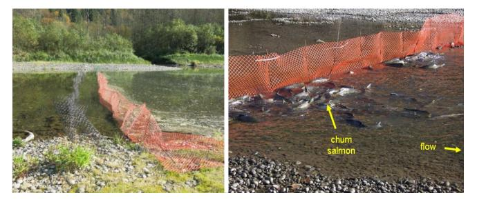
Figure 17 Exclusion fencing installed on the Herrling Island Side Channel in its initial (right panel) and more advanced progression (left panel) (Source: Living Resources 2013).
