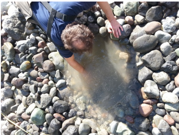
Photo 1: Excavating sediment for sediment trap installation.
