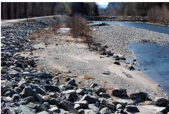
Typical riprap bank protection with adjacent bar displaying sparse shrub
