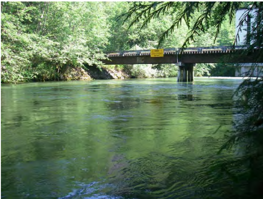
Photograph 18: View of Site 10 looking upstream from RUB during high flow must-run, June 4, 2009.
