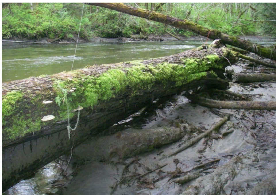
Photograph 22: Partial flow at Site 11 during power generation ramp-down, view from RUB looking upstream, May 6, 2009.
